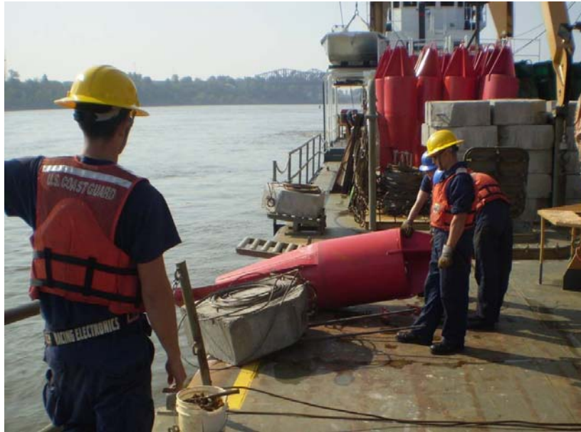
Figure B-3. Crew ready to set buoy using pinch bars to launch sinker.
