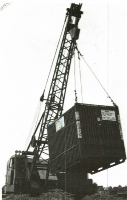
HOISTING CONEX CONTAINER FOR CONVOY LOADING
