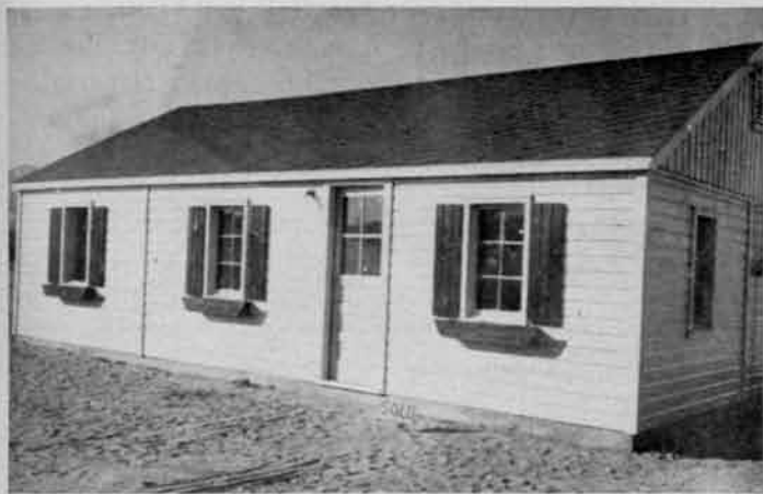
Completed Prefabricated House. Four days—3½ Hours after arrival of materials.
