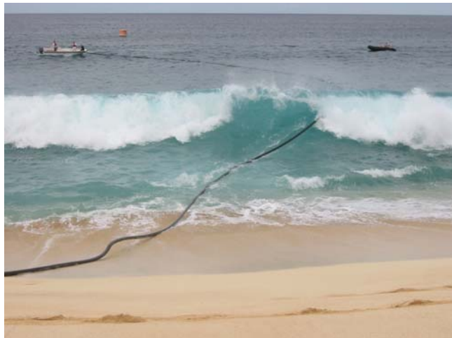
Figure 8. Deploying Borehole Liner Over Sand
