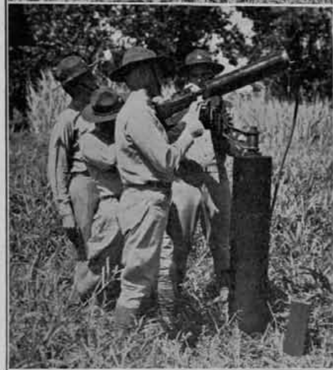
The railway rail type (above) and the reinforced concrete type (below) of improvised fixed mounts.
