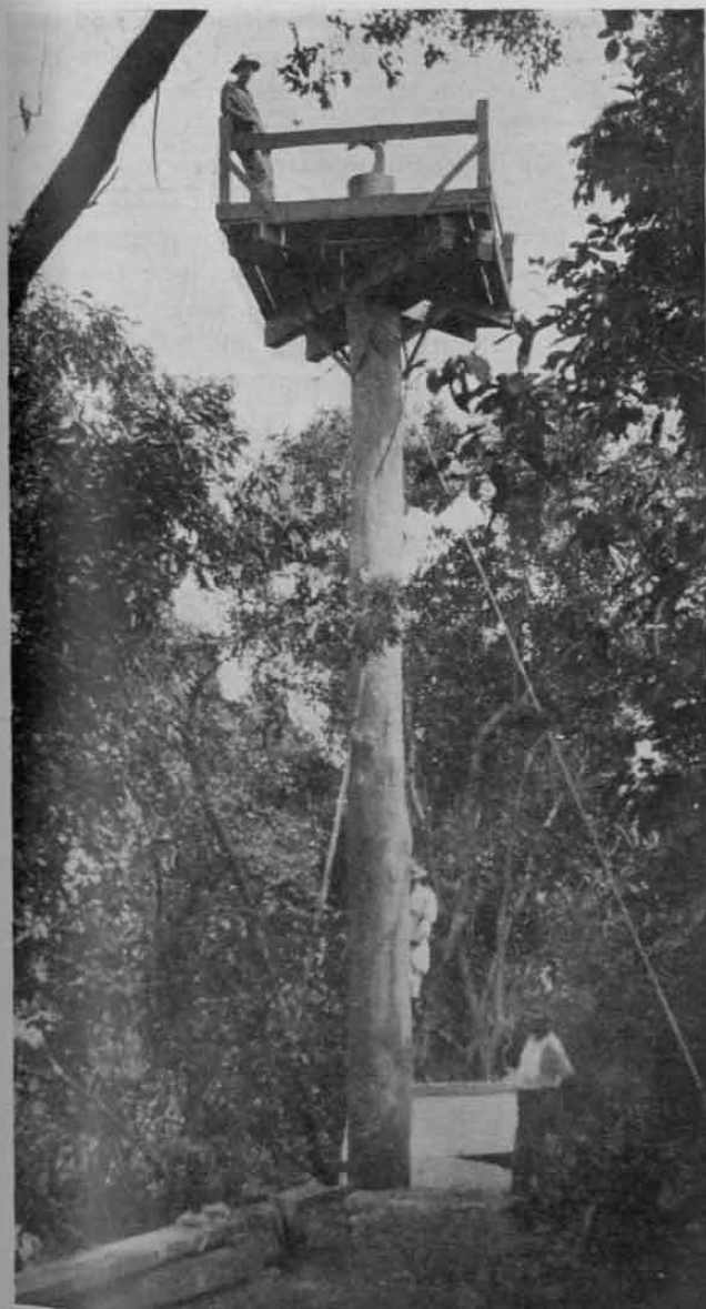
Poles, guys and platform are clearly shown here.
