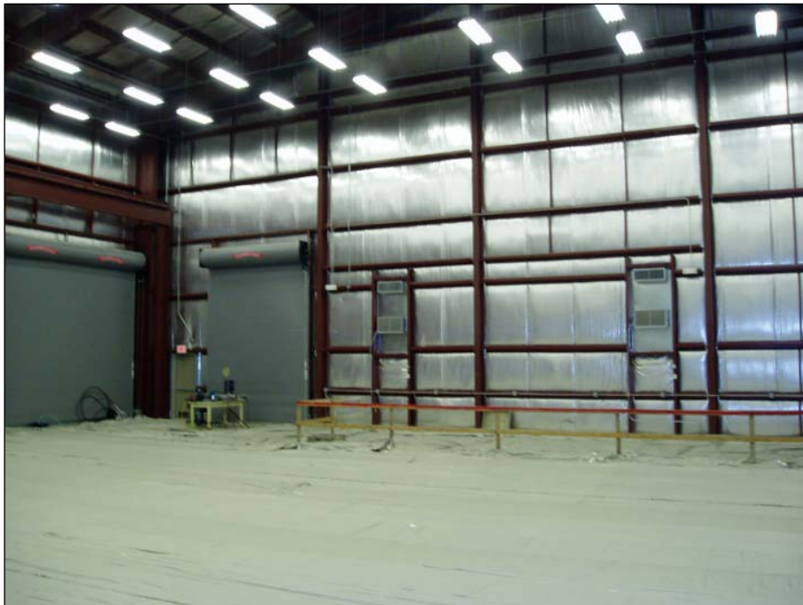
Figure 5-4. ERG Building Interior with Covered Floor
