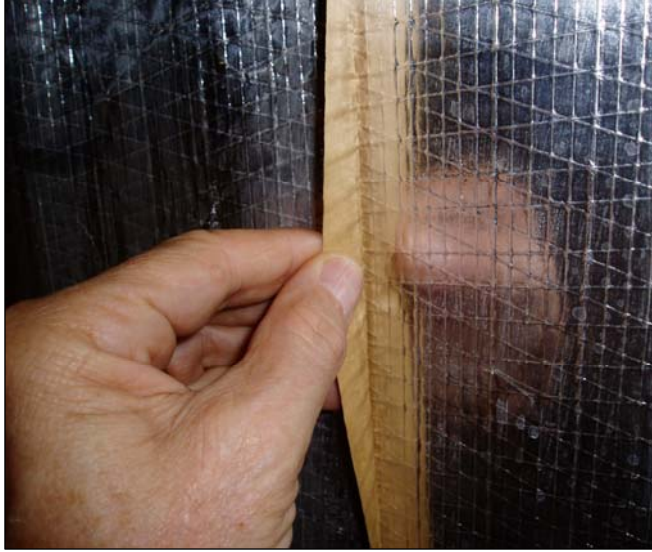
Figure 5–8. Noncontacting Overlap Between Insulation Sheets
