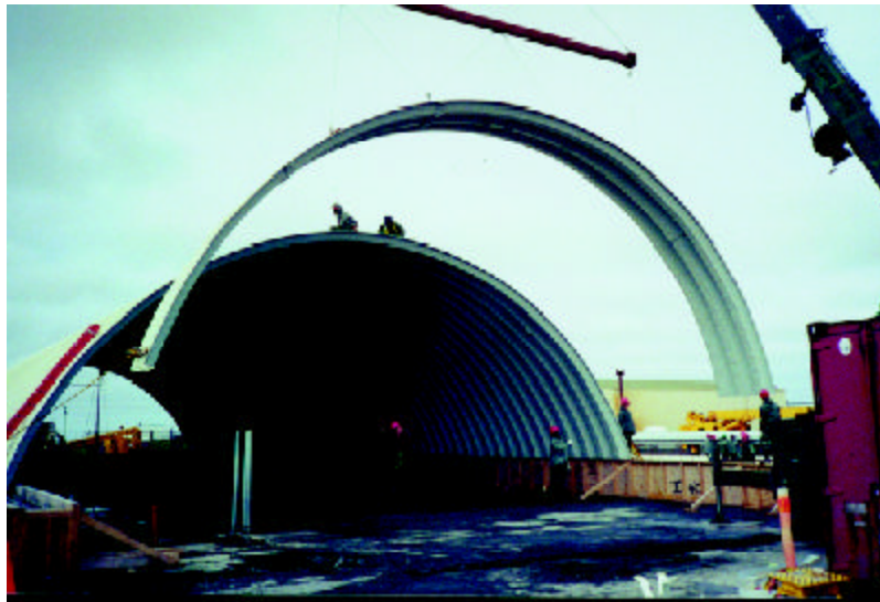
A crane lowers panels into place during RED HORSE construction of a Super K-Span building at Naval Air Station Keflavik, Iceland. (Photo courtesy 203rd RHF)
