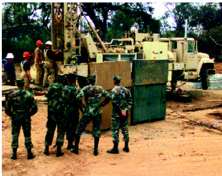
(Right) TSgt Mike DeShon, NCOIC of well drilling for the 819th RHS, explains the operation of the SS-135 drilling machine to Brig Gen Earnest O. Robbins, who visited the New Horizons '99 team in June. The 1,049-foot well was the first solar-powered well in U.S. military history. (Photo by TSgt Scott Wagers)
