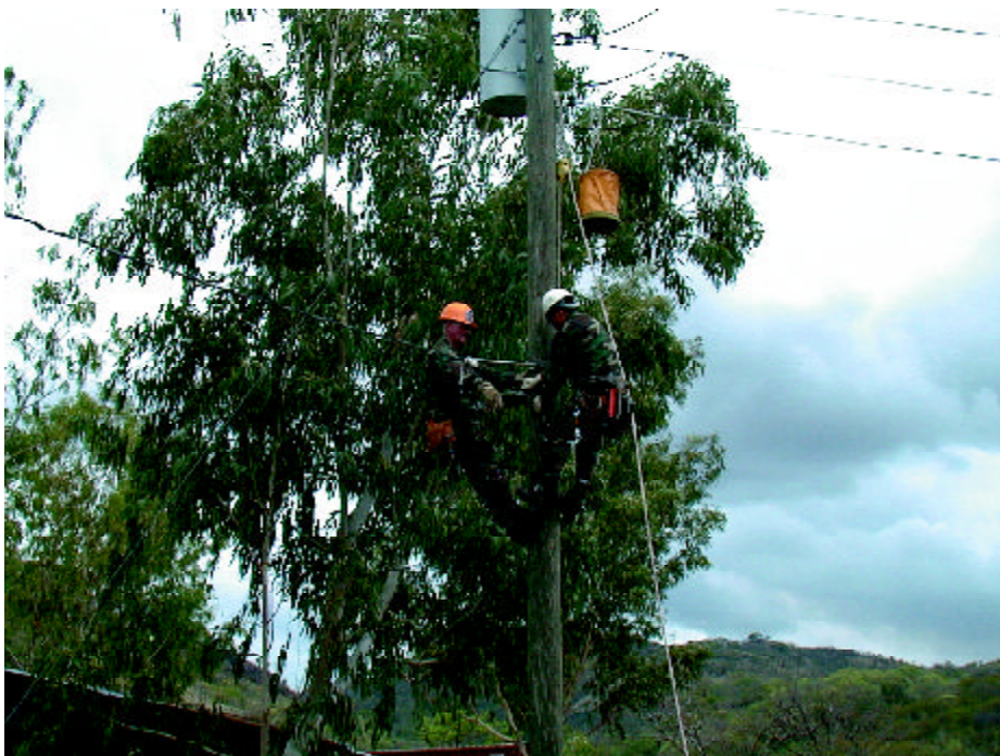
SMSgt Tommy Guerra, 144th CES, and SSgt Rex Rekow, 142nd CES, install a secondary feeder to the billeting area as part of the complete rewiring of the secondary distribution system for the base camp.
