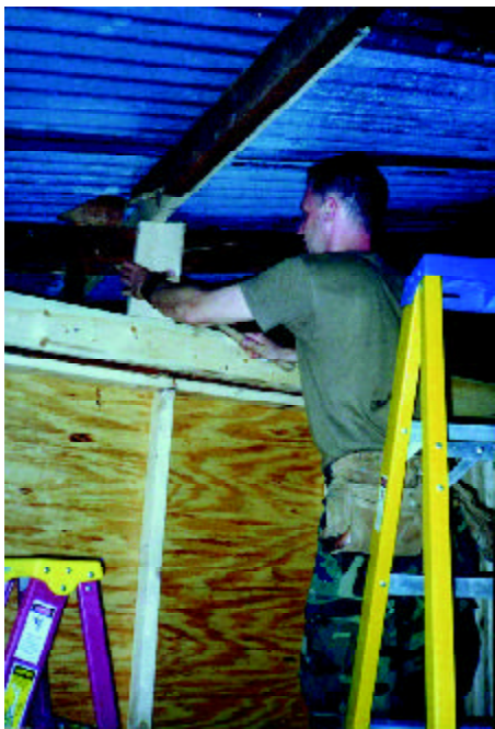
MSgt Chris Bryant, 142nd CES, repairs a termite-damaged roof purlin in the chapel. There was extensive termite damage to the wood structures at the base camp.
