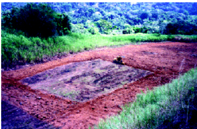
Remote subsurface plowing of airfield target. (Photo by Larry Johns)
