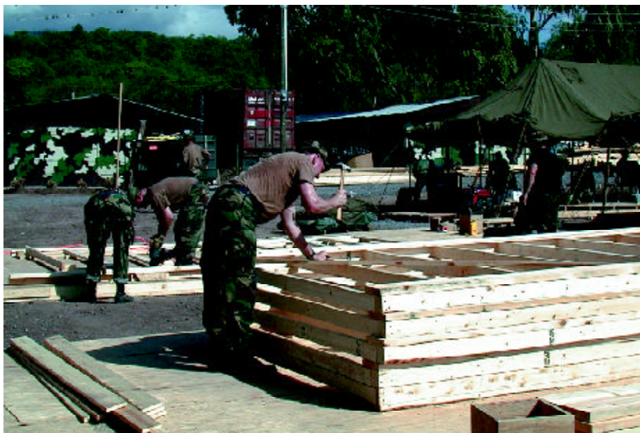
Prime BEEF members construct modular tent floors for transport to a forward base camp. (Photos courtesy 142nd CES)
