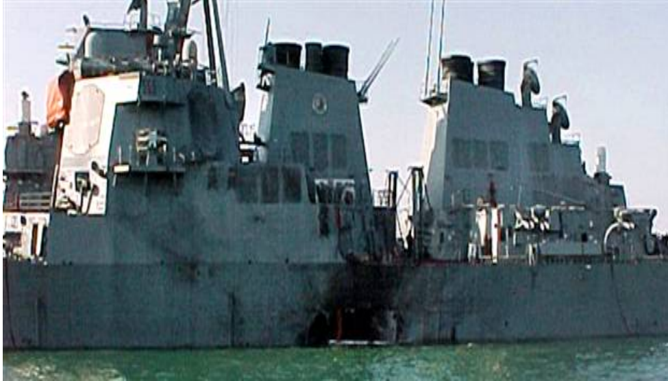
Figure 2. Additional View of Damage to USS Cole 33
