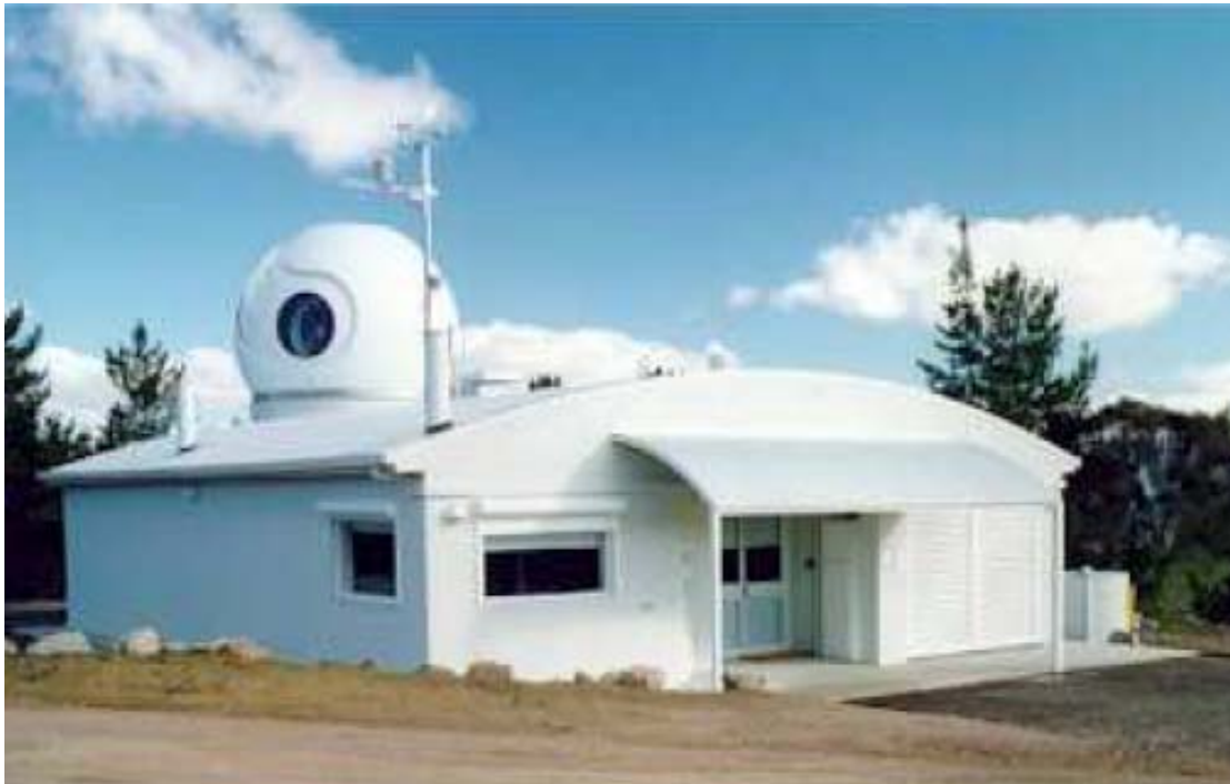
Figure 35. A Satellite Tracking Electro-optical System
