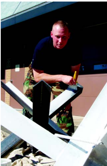
SSgt Alan Vanguilder, 148th CES, Minnesota Air National Guard, paints one of several newly constructed “road jacks” Oct.1. The Wing’s CEs constructed numerous jacks for use on roadways to provide enhanced protection for the resources and personnel supporting Operation NOBLE EAGLE. (Photo by MSgt Dean V. Kuhlman)
