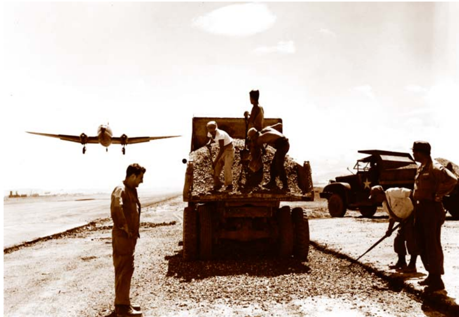
Members of the 811th EAB barely take notice of a C-46 Commando coming in for a landing as they work on a runway overrun.
