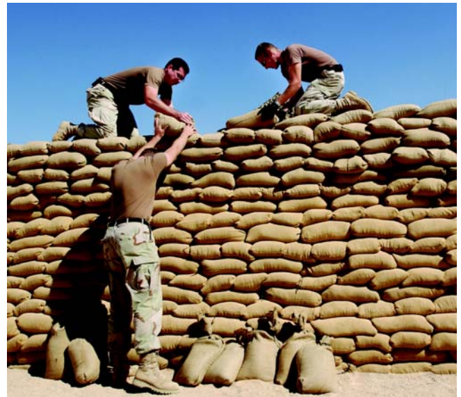
405th Air Expeditionary Wing firefighters add sand bags to a security wall at a deployed location Jan. 5. (Photo by SSgt Shane Cuomo)
