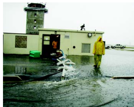
(From top to bottom) Approximately 3 feet of water stood in the basement of the West Airfield vault when the top photo was taken and 4 feet when the second photo was taken. David Washington (in doorway) and SrA Andrew Diehl, both from the 12th CES, at Randolph's West Airfield Vault. Approximately 30,000 gallons was pumped out of the basement that day. (Photos by MSgt Luis A. Adams)
