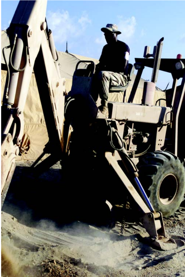
A CE staff sergeant excavates a trench so that drainage pipe can be laid at an undisclosed forward operating site Nov. 18. (Photo by MSgt Thomas Cook)
