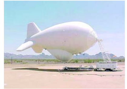
The Civil Engineer Division is currently working an initiative to standardize the Tethered Aerostat Radar System fleet and mooring systems. Here, the TARS Aerostat is moored on a launch pad at Deming, NM. (Photos courtesy PMS/CE)
