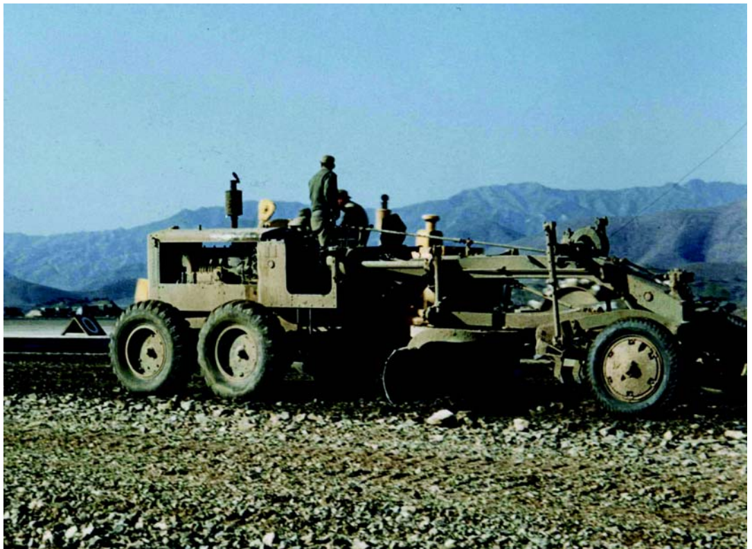
Rare color photograph of civil engineers in Korea. Runway grading at K-55 (Osan AB), 1952.
