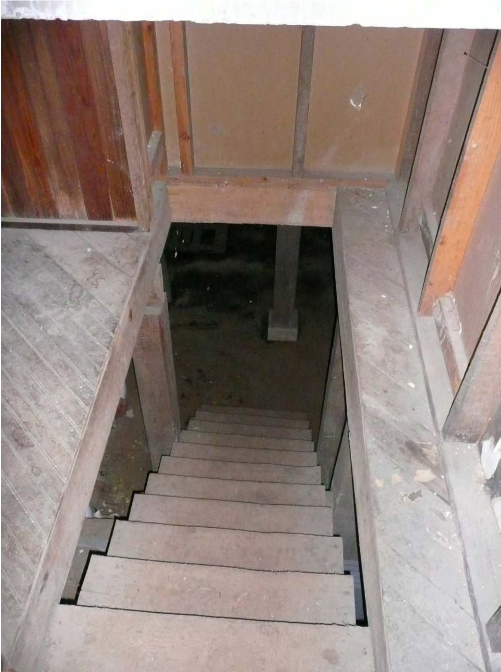
Photo 35 – view of wood stairs leading to the basement
