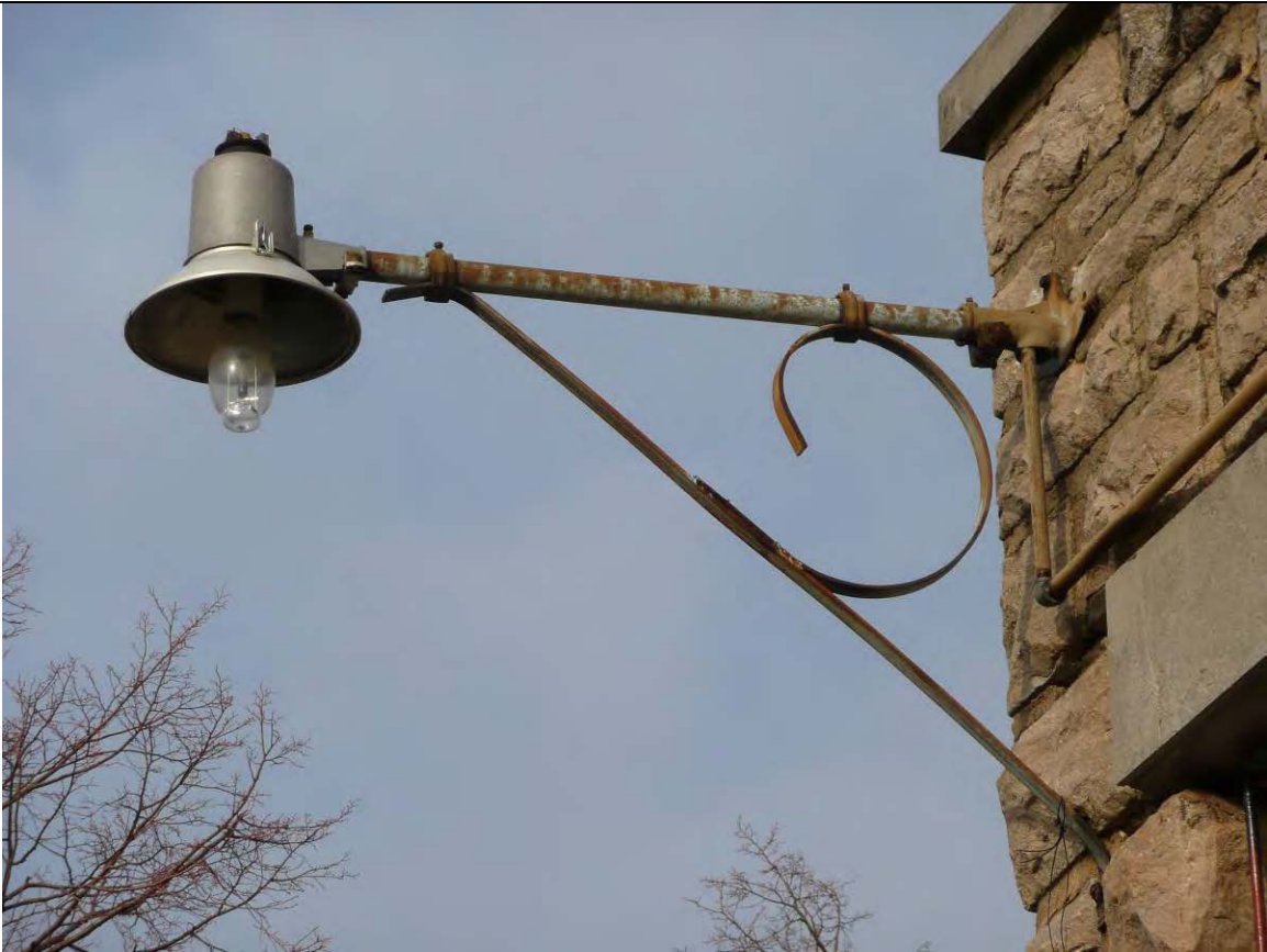
Photo 8 – detail of original light fixture on the south elevation
