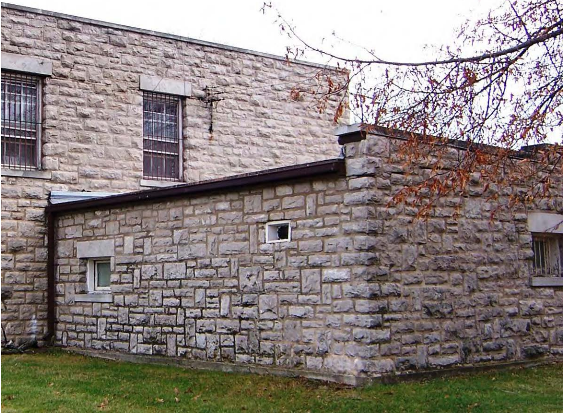
Photo 27 – parapet detail on west elevation of one-story garage
