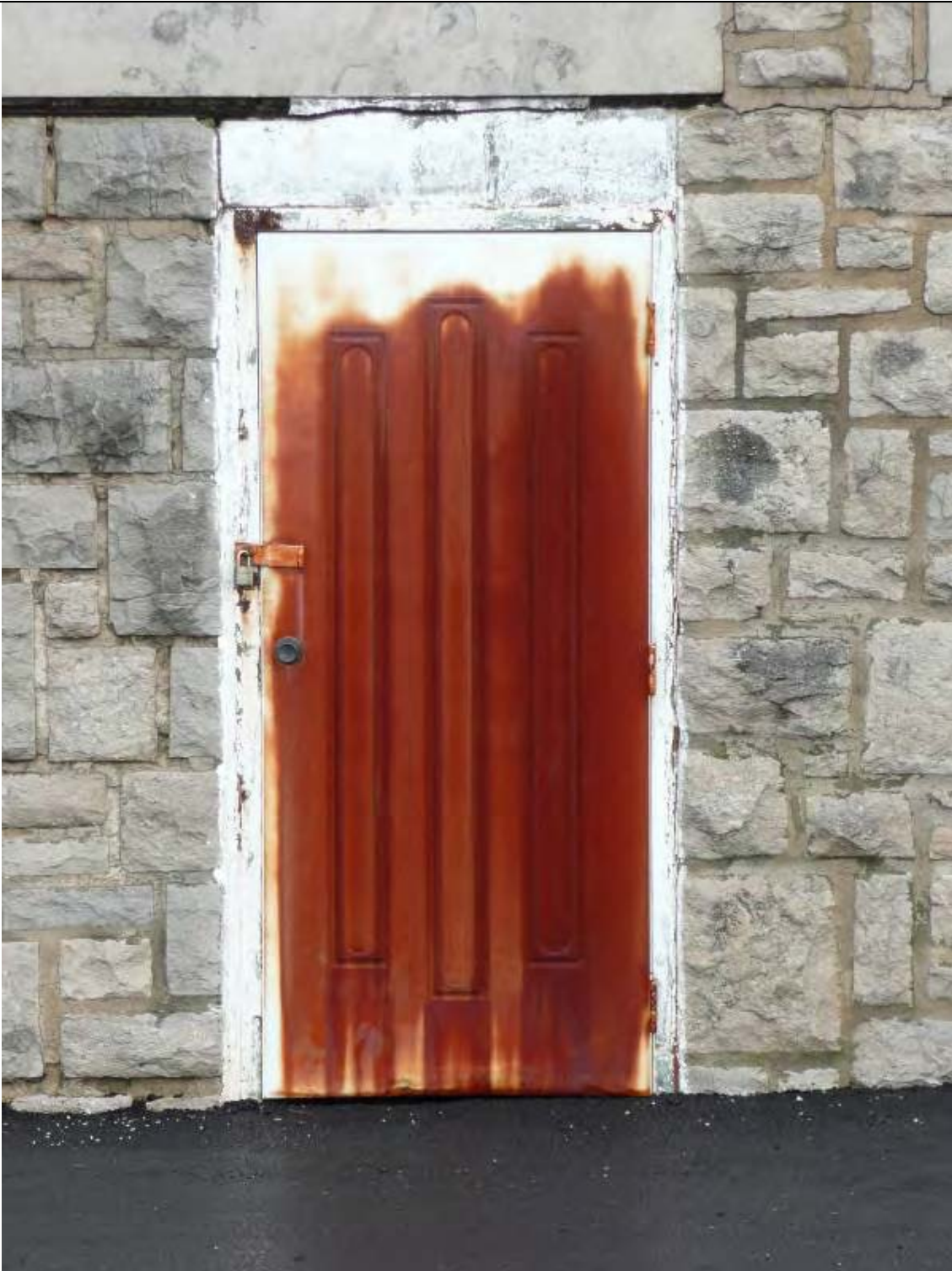
Photo 18 – metal entry door into garage
