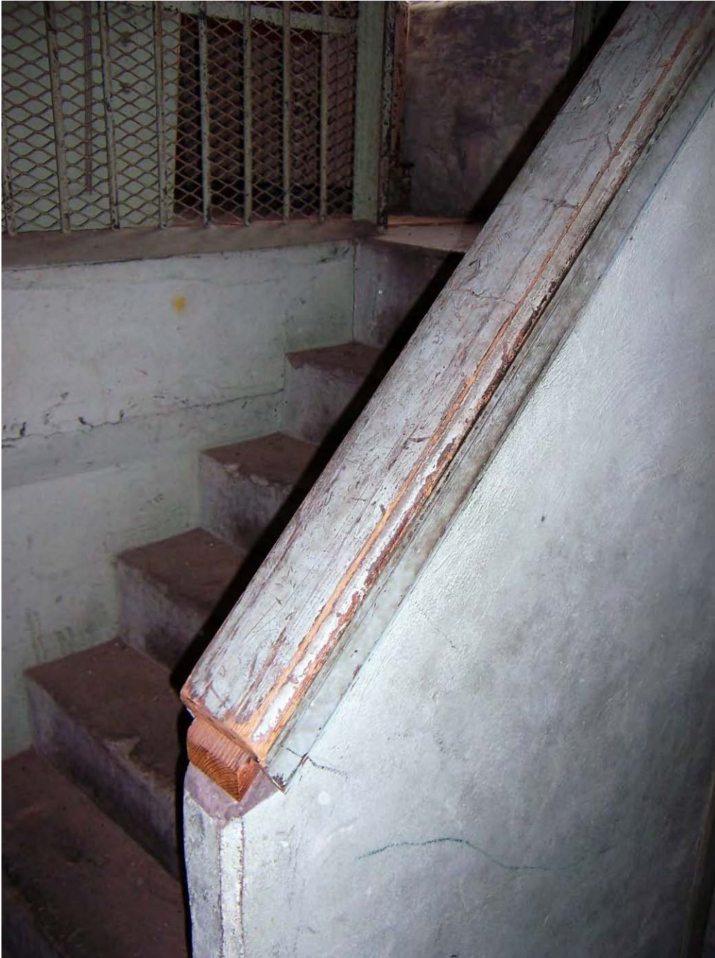
Photo 37 – detail of handrail on stairs leading to the second floor
