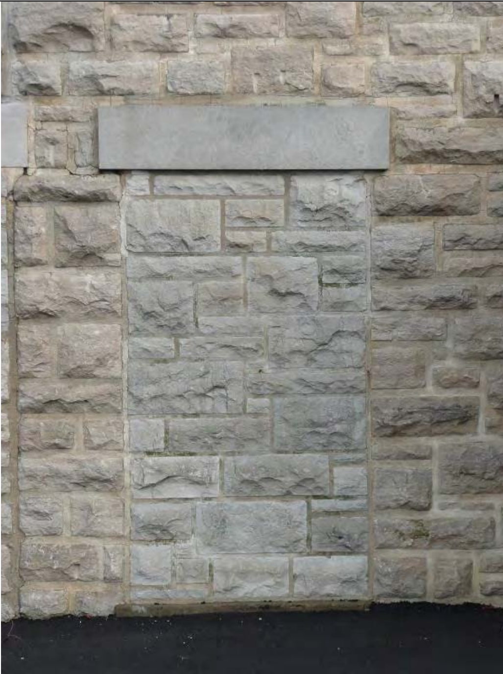
Photo 4 – view of modified filled window opening on south elevation
