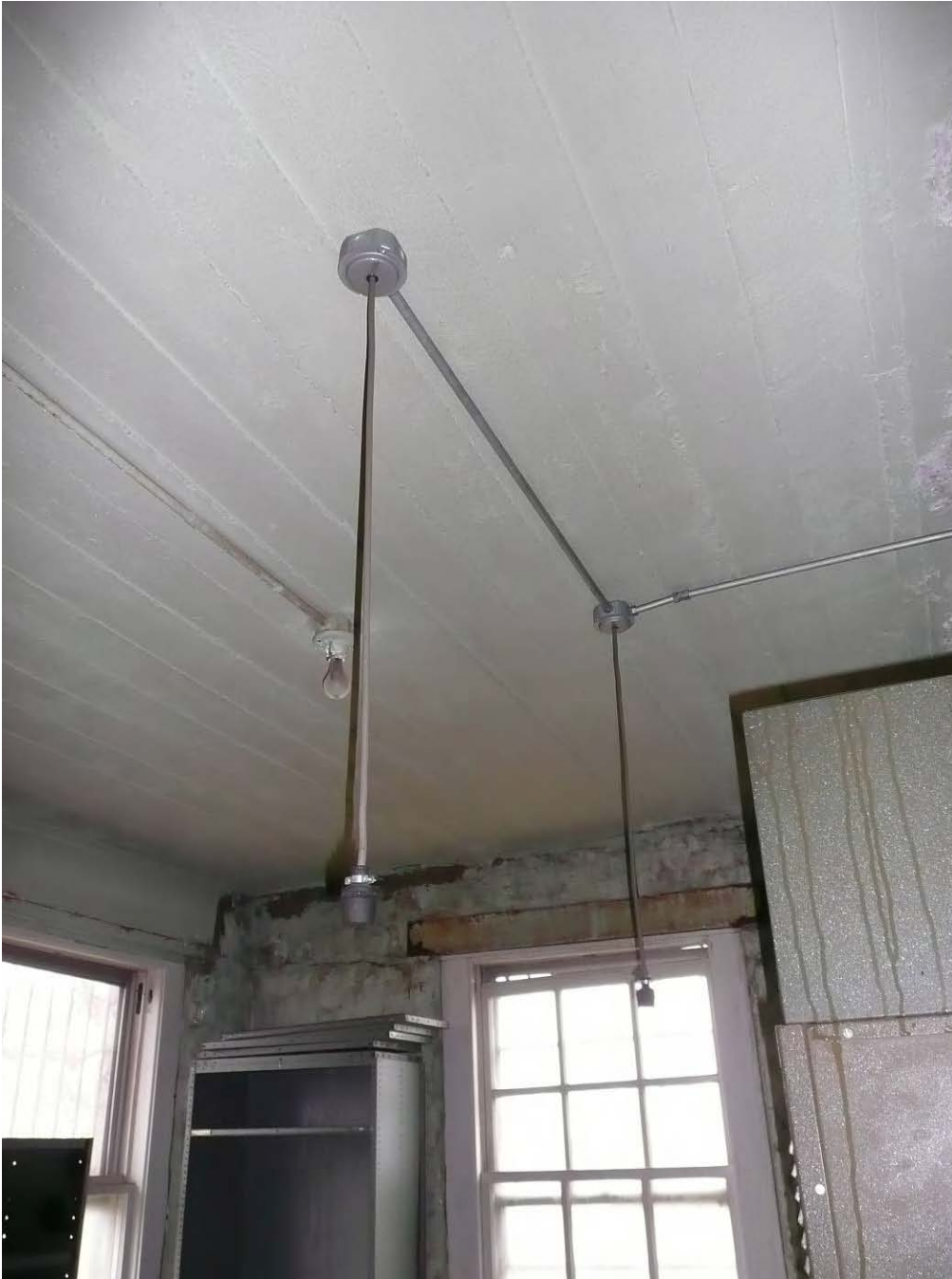
Photo 39 – view of concrete ceiling
