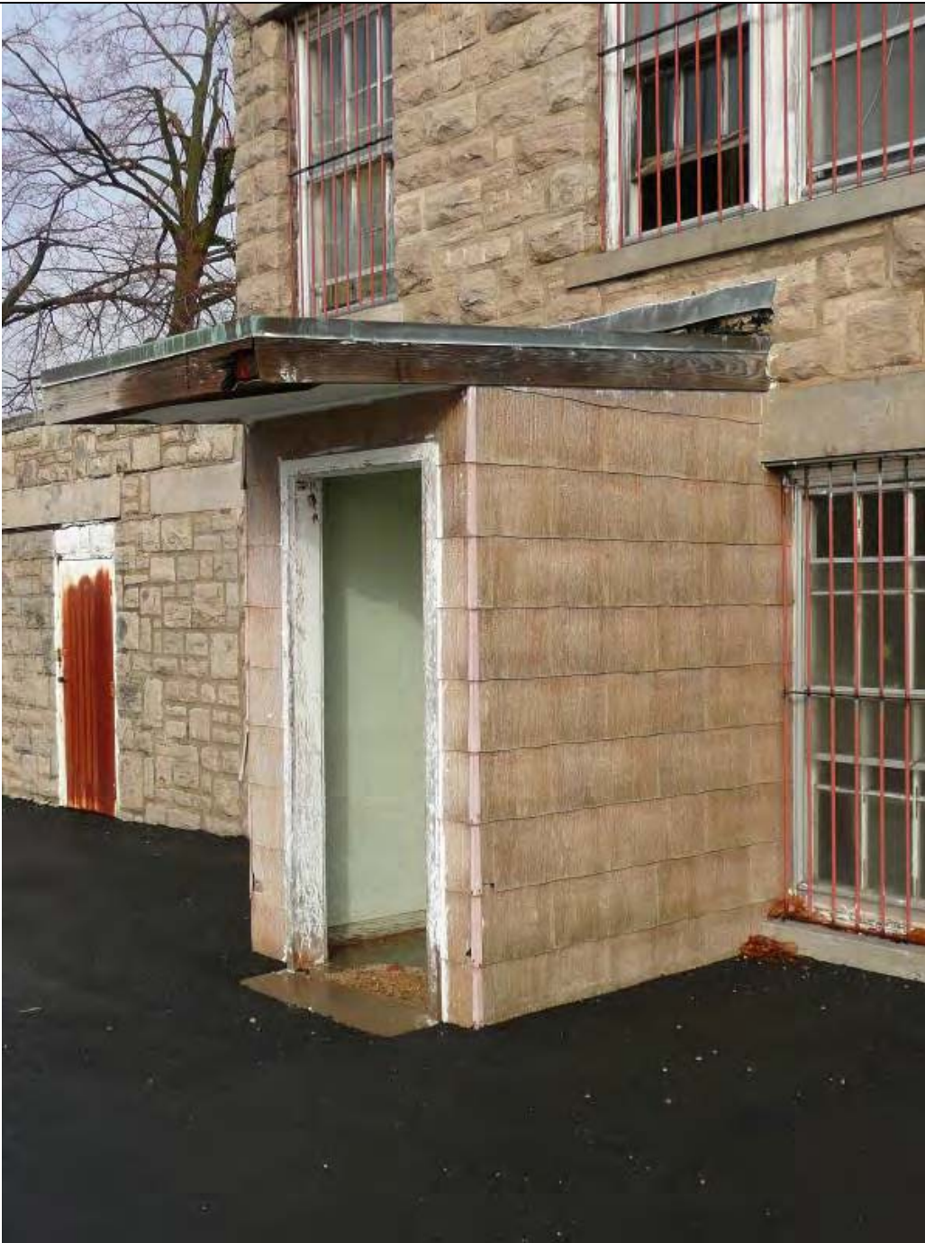
Photo 5 – close-up of vestibule addition on south elevation
