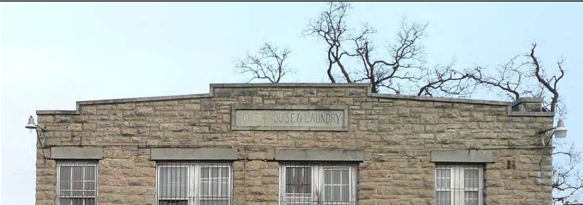
Photo 28 – stepped parapet detail on south elevation
