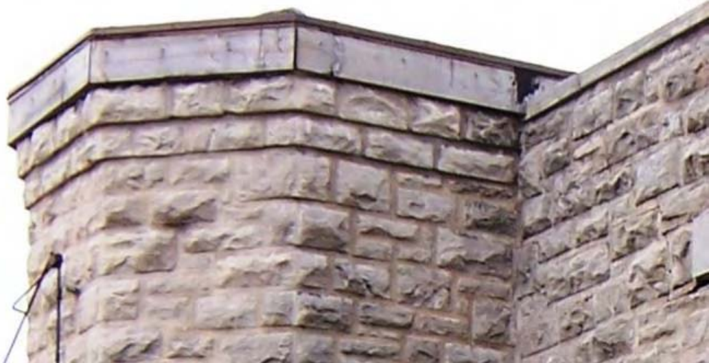
Photo 10 – close-up of chimney stack modification
