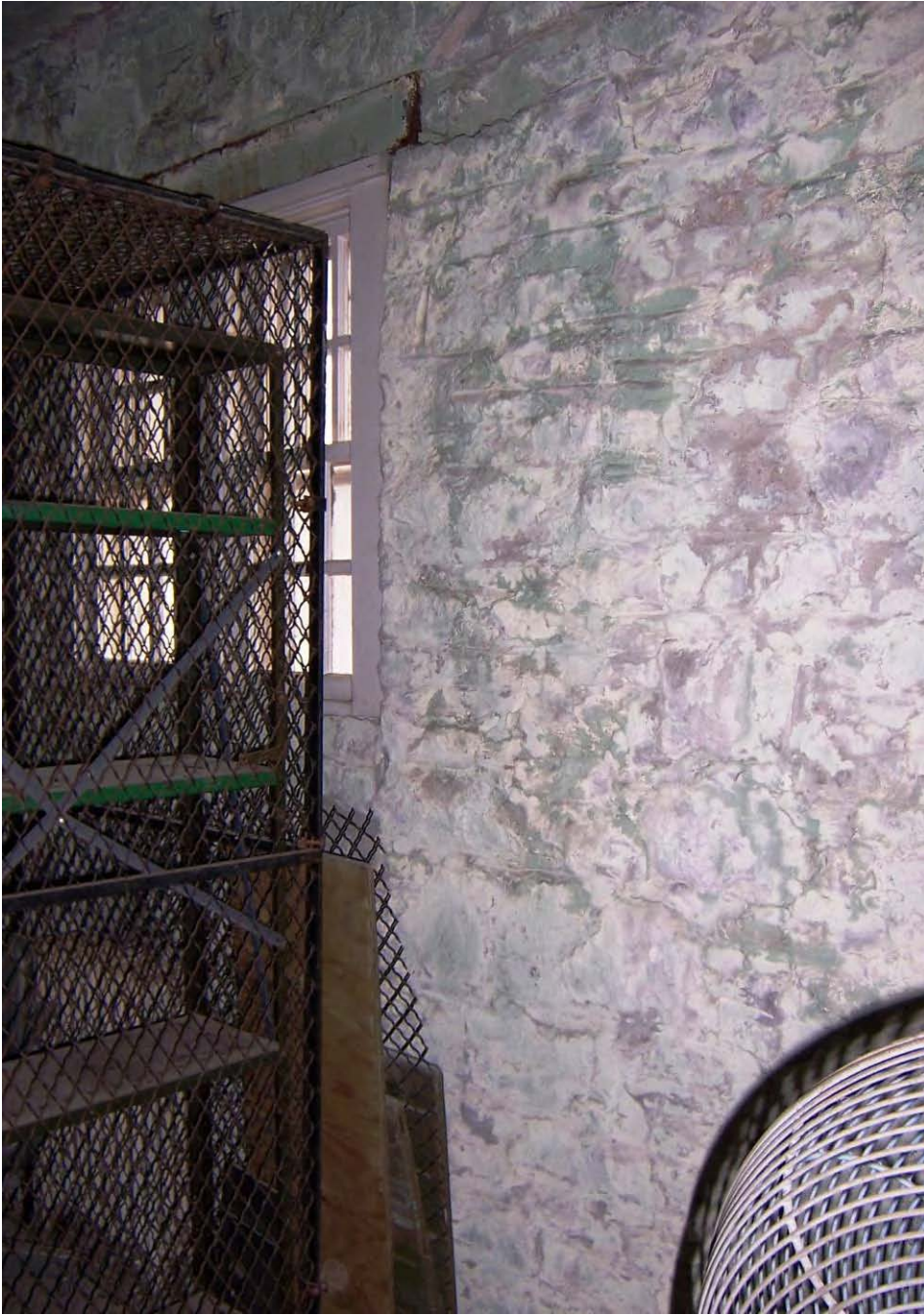
Photo 38 – interior view of cut limestone wall
