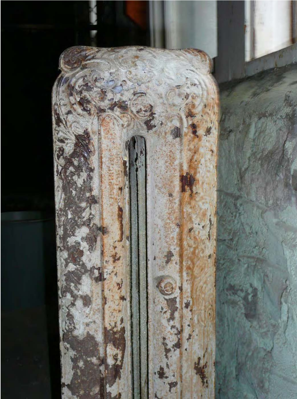
Photo 43 – example of original radiator on second floor
