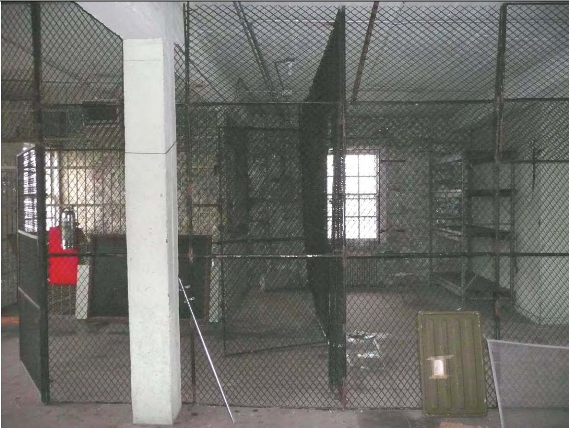
Photo 34 – overall interior view of the second floor
