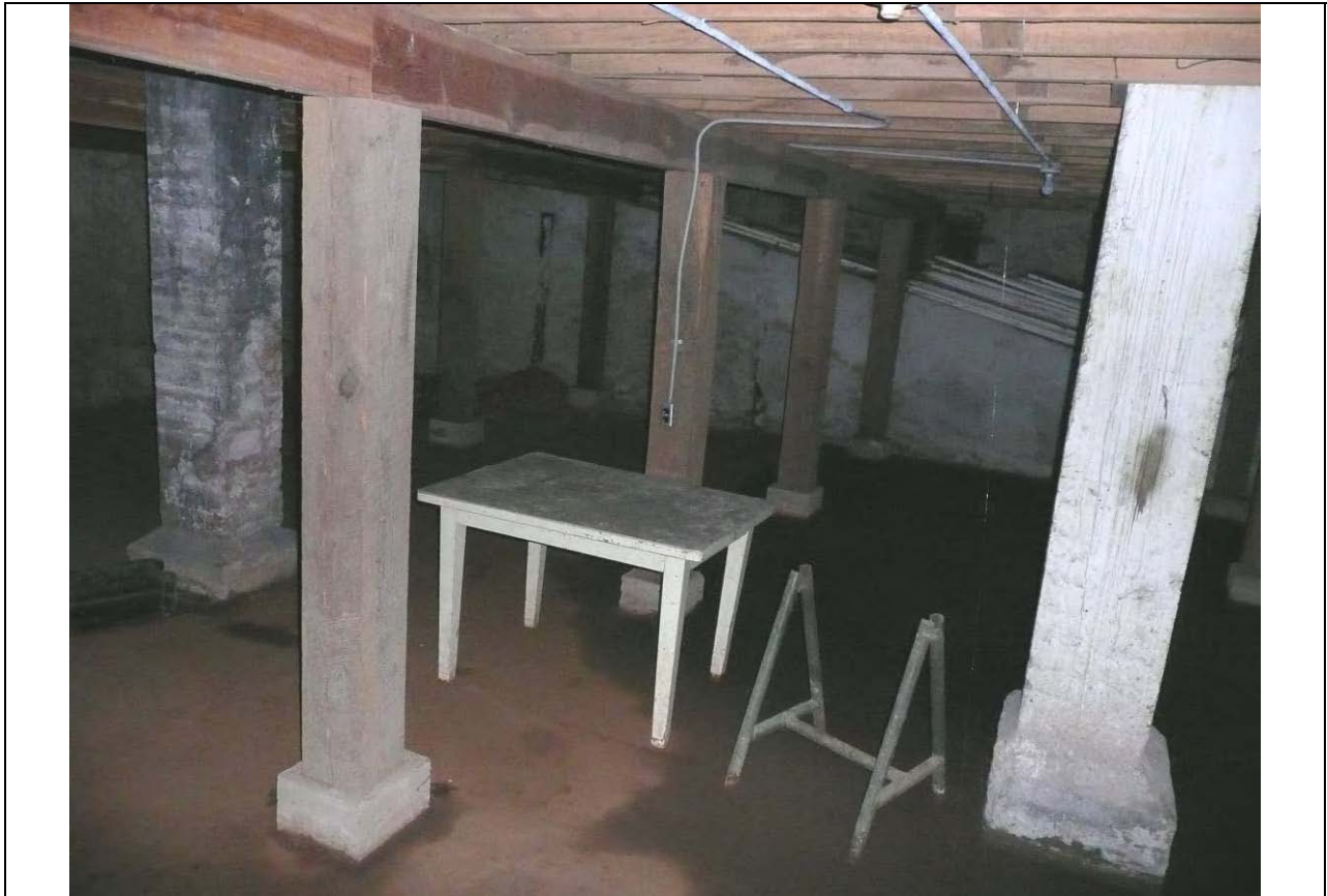
Photo 15 – view of added wood columns used to support first floor
