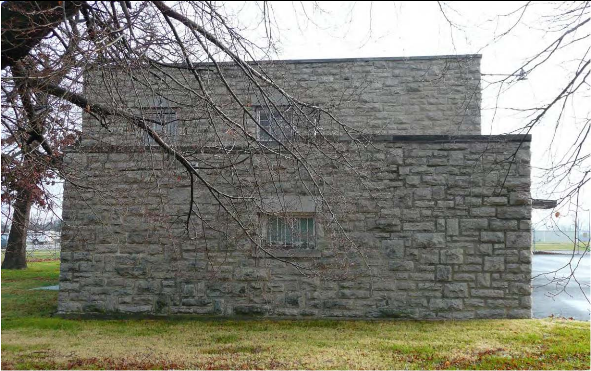
Photo 13 – west elevation; overall view
