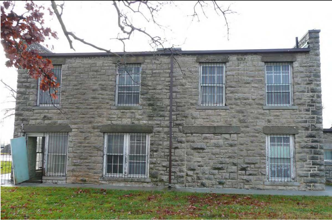
Photo 11 – left side of the north elevation; overall view
