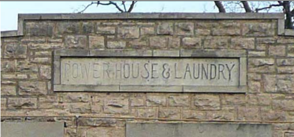
Photo 7 – detail of "POWER HOUSE & LAUNDRY" etching
