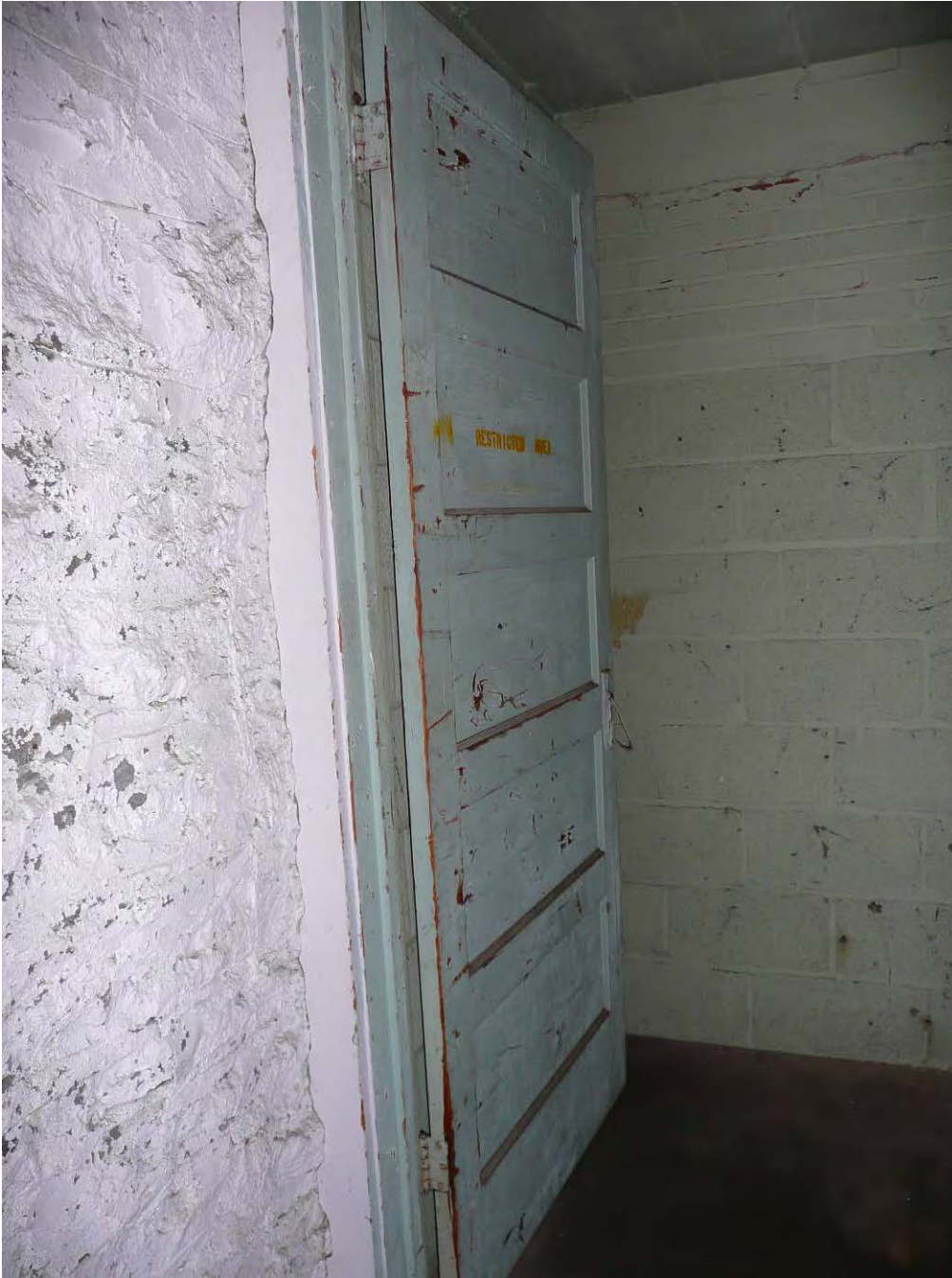
Photo 40 – view of five-panel wood interior door and door opening filled with concrete masonry units
