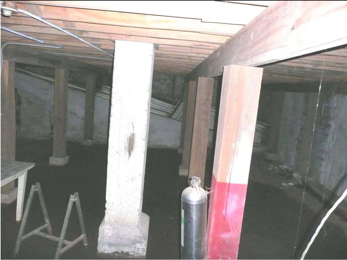
Photo 29 –interior view of basement
