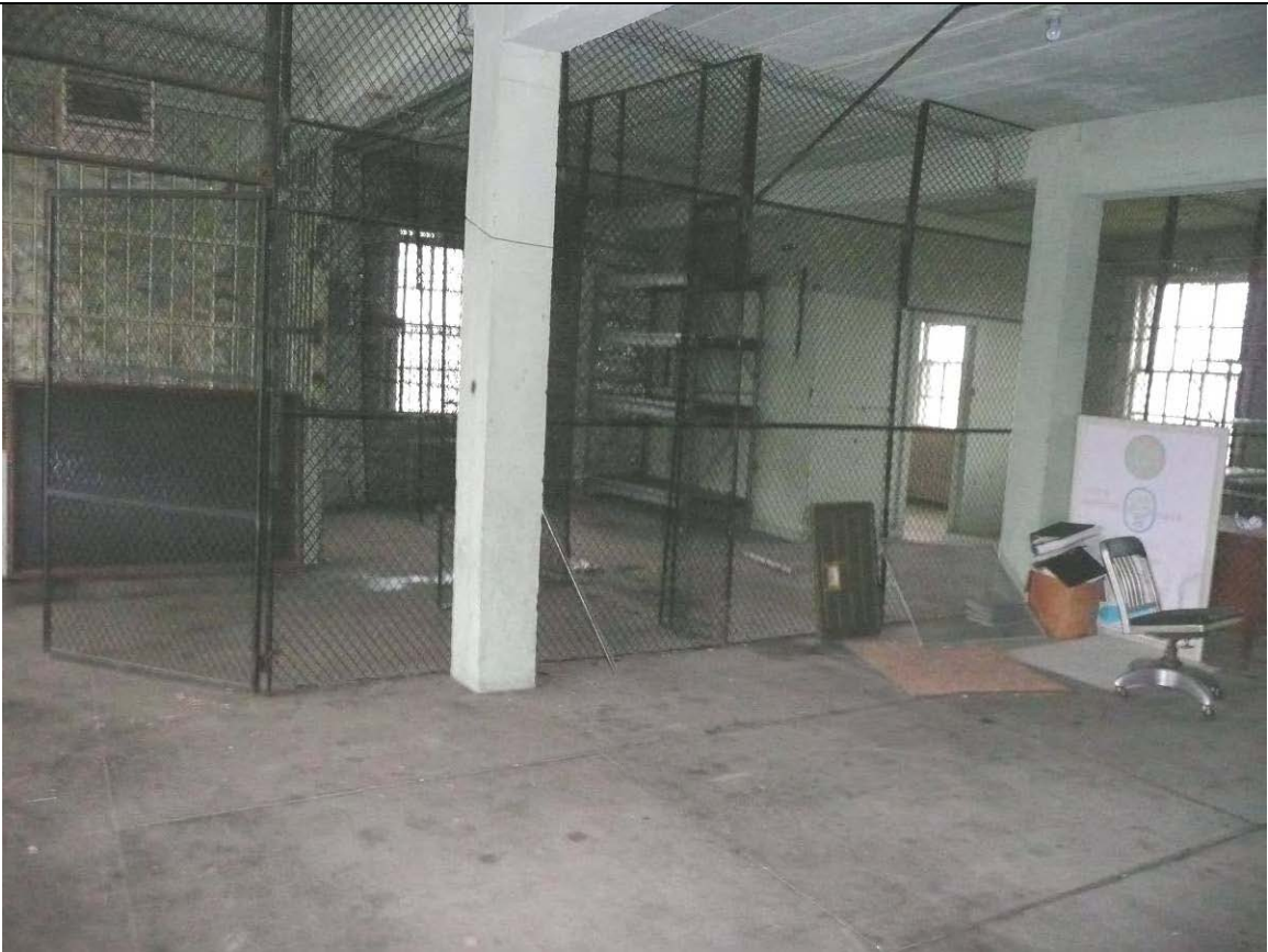
Photo 14 – interior view of two continuous concrete columns on second floor
