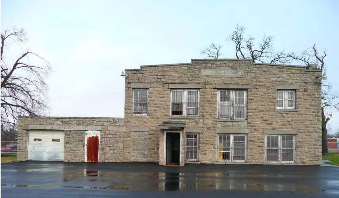
Photo 1 – south elevation; overall view
