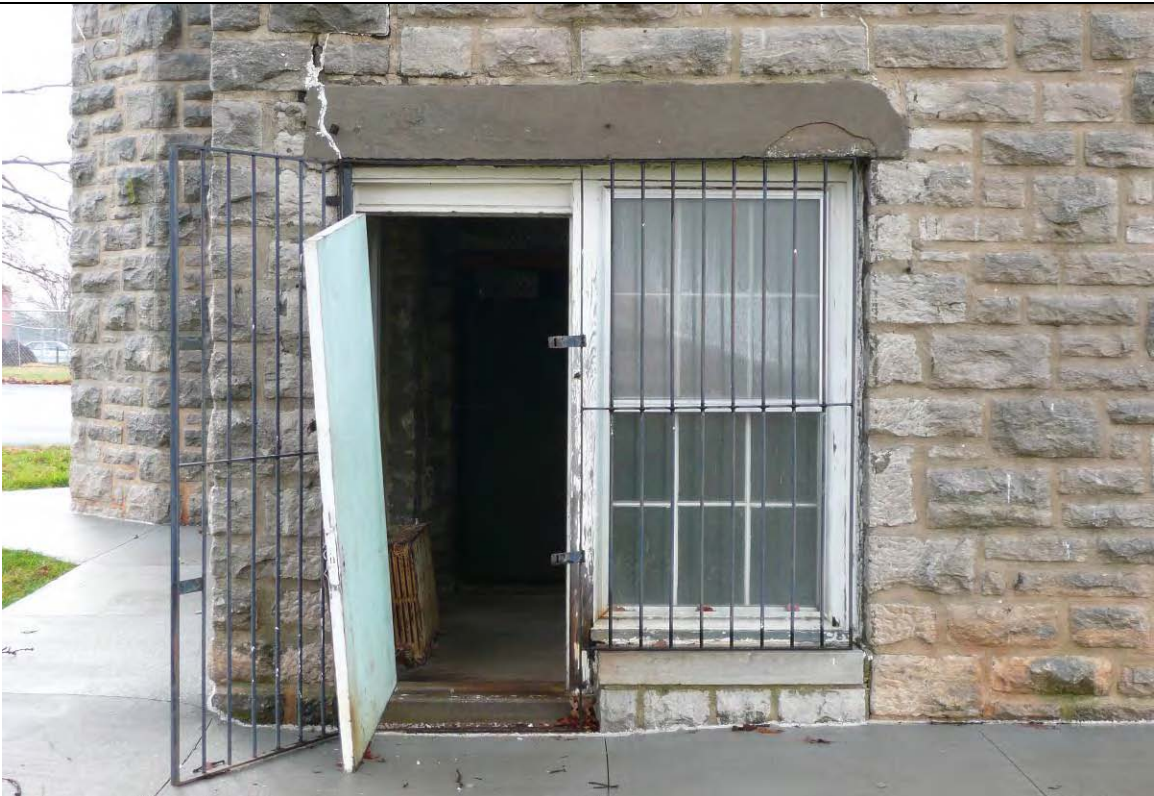
Photo 12 – close-up of window modification on north elevation
