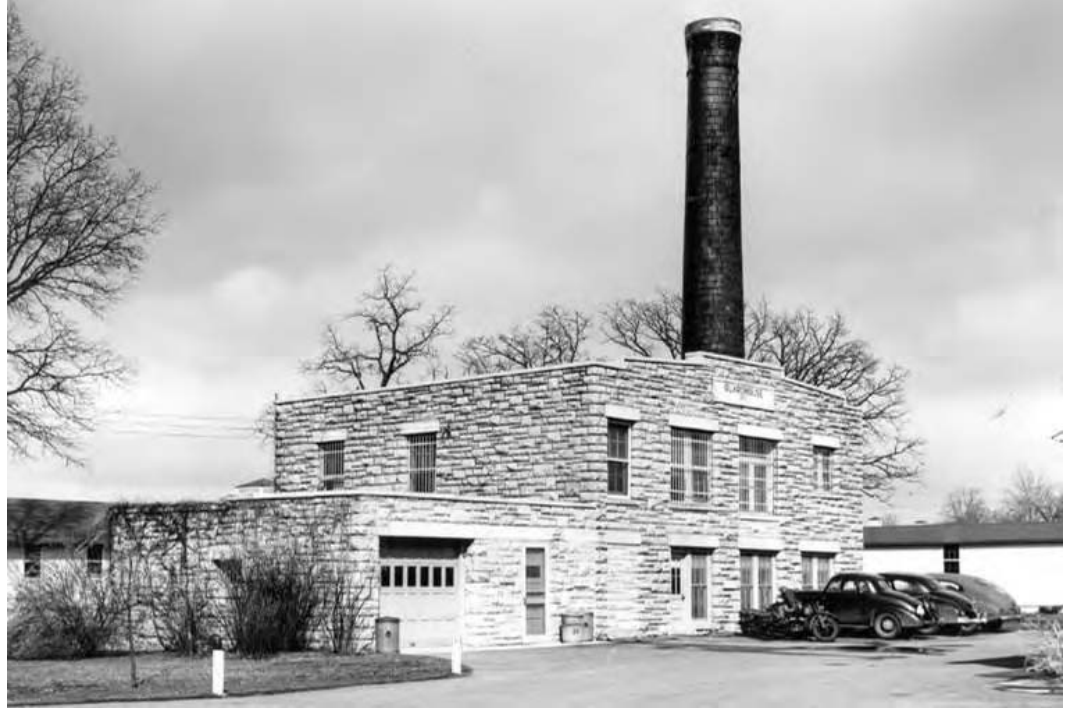
Figure 4. O'Reilly General Hospital Guardhouse, 1942 (courtesy Springfield-Greene County Public Library).
