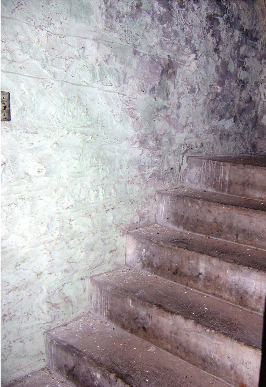
Photo 36 – view of switchback concrete stairs leading to second floor
