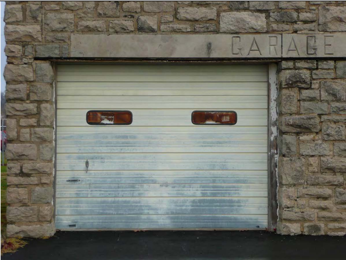
Photo 17 – replacement metal garage door on south elevation
