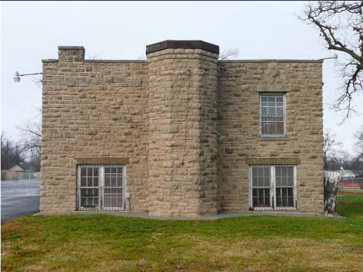
Photo 9 – east elevation; overall view
