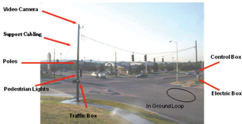
Figure 6-6. A Typical Signalized Intersection
