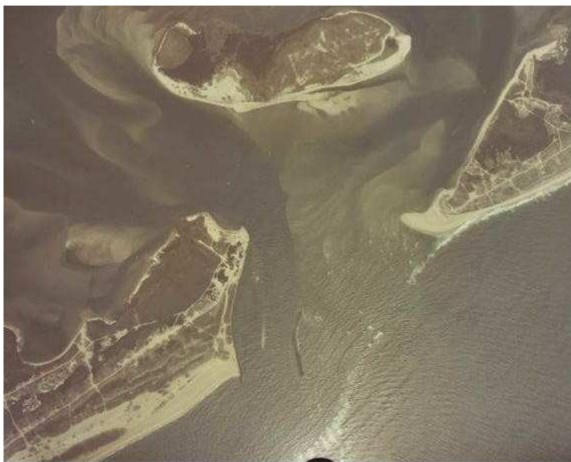
Fig. 12. Breach at Moriches Inlet, New York, September 21, 1980. Photograph taken 9 months after the January 1980 breach. Note east jetty became isolated from land because of the breach.
