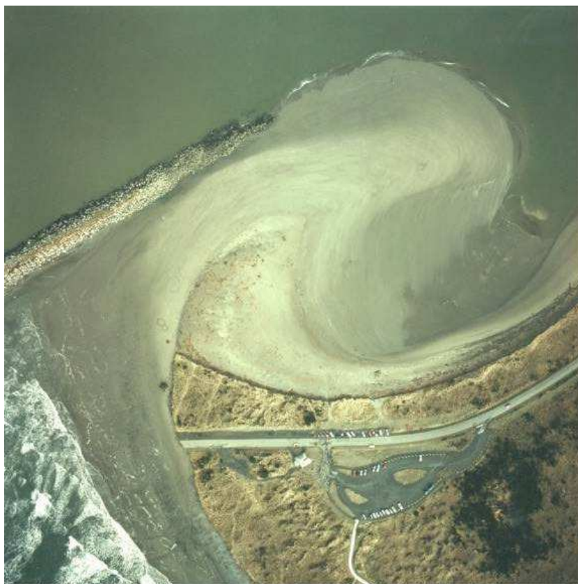
Fig. 3. Breach at south jetty of Grays Harbor, February 1994, 2 months after inception.
