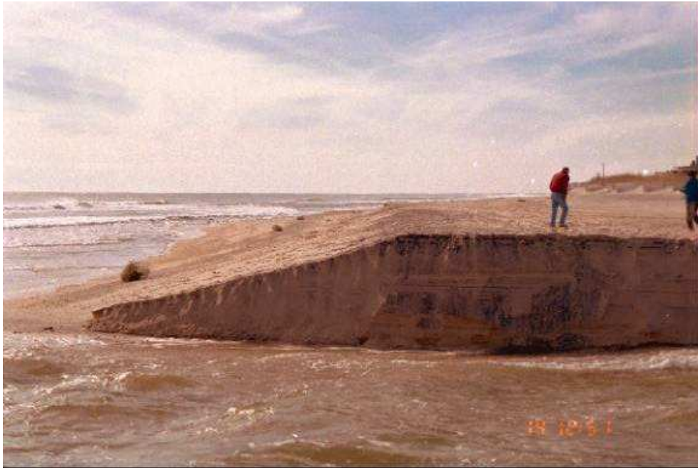
(a) Looking west at breach cut through beach berm at Mecox Pond; Atlantic Ocean to left.
