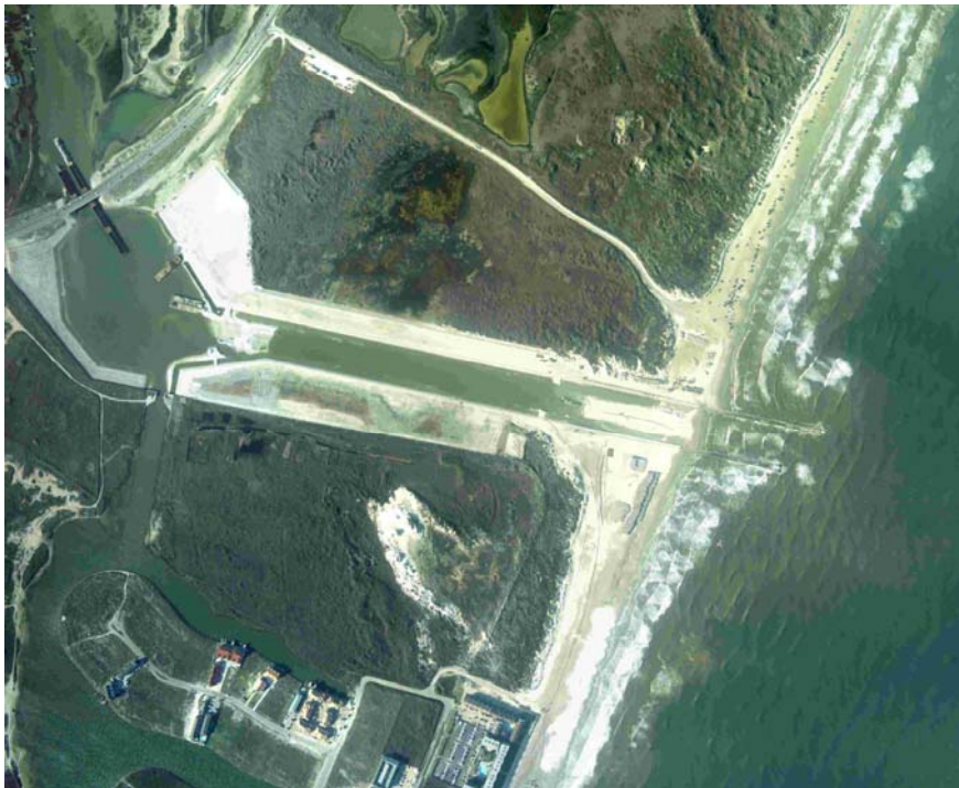
Fig. 2. Packery Channel (Inlet), Texas, under construction, March 2005
