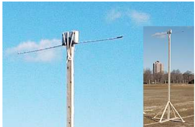
Fig. 3. Node B mounted on a wood tower. The antennas are mounted on horizontal, 3ft long masts
