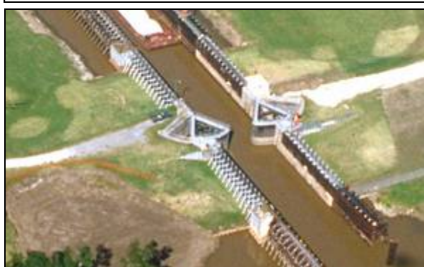
Illustration 7. Plan diagram of sector gate operation (top) and aerial view of lock with sector gates (bottom).
