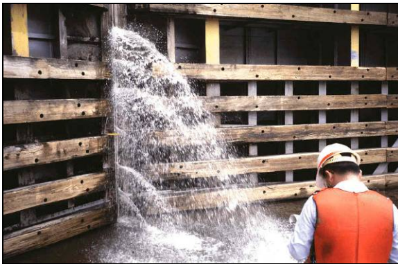
Illustration 4. Downstream miter gate.
