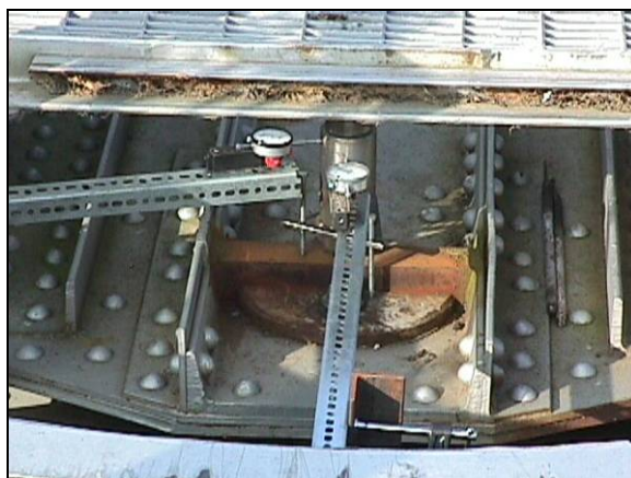
Figure 5. Preparations for measuring bushing wear around axis of rotation.
