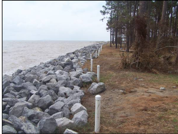
Figure 13. Bank line revetment structure.
