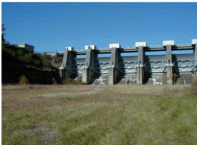
Illustration 25. View upstream at a dry spillway.
