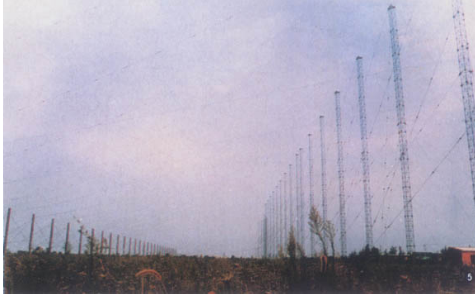
Figure 18. The Transmitter Antenna Element of Surface Wave OTHR (From [20])
