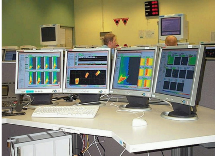
Figure 14. An Interior View of the JORN Coordination Center (From [16]).
