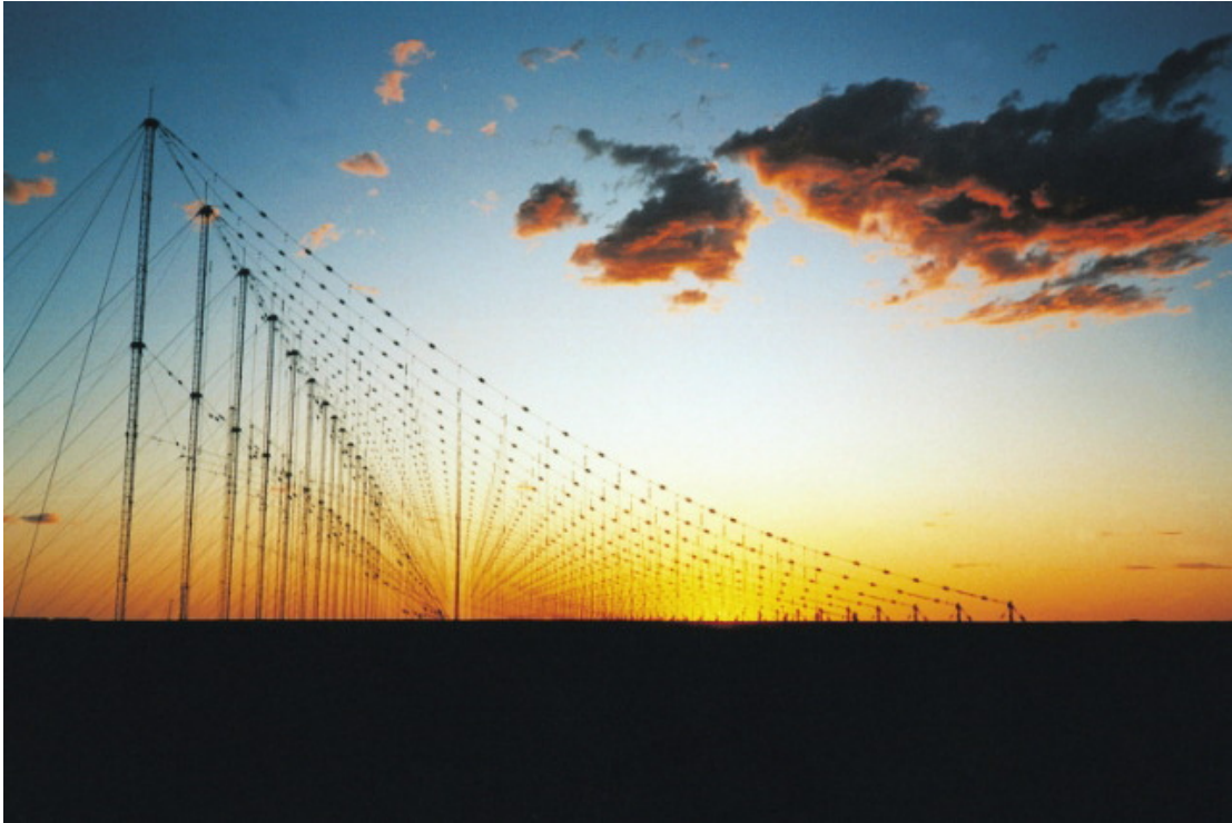
Figure 12. The JORN Transmission Antenna Array (From [15]).
