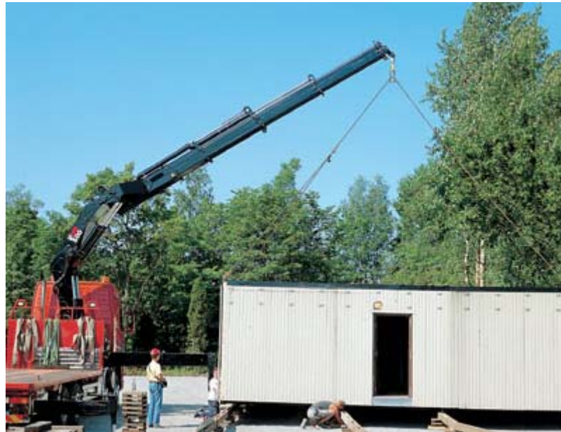
Figure 17: Hiab 500 Truck Mounted Crane
