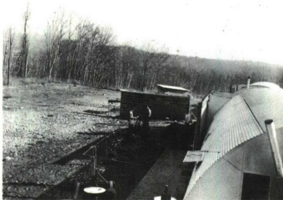
Figure 6 - 1500-lb oxygen-alcohol motor-firing facilities
