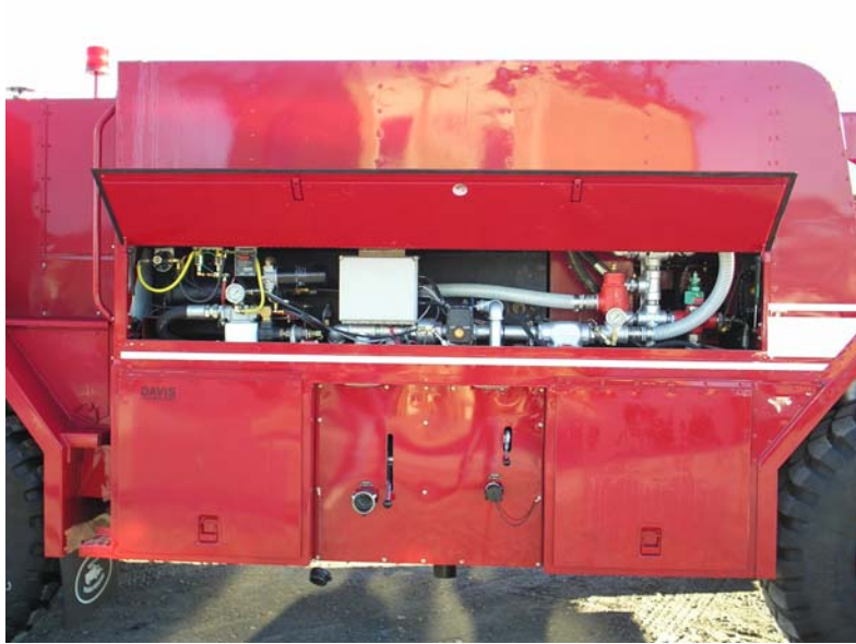
Figure 3.3.10: The UHP P-19's driver's side plumbing.
