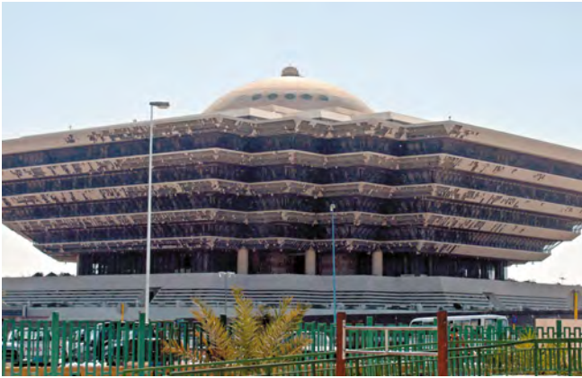
The Ministry of the Interior was damaged by an explosion when terrorists launched coordinated car bombings and battled security forces in Riyadh on December 29. (AP Photo/STR)
