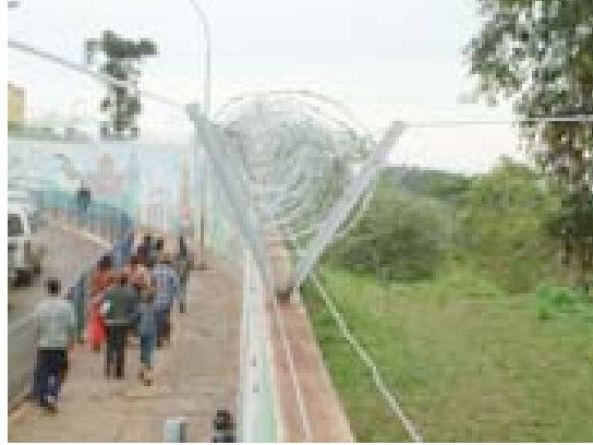
Figure 2. Security Barrier with barbs (harpoon style), installed by Brazil to prevent the sacoleiros from throwing their merchandise in the river, from which others later collect it, thus bringing it into the country and mocking control measures.
