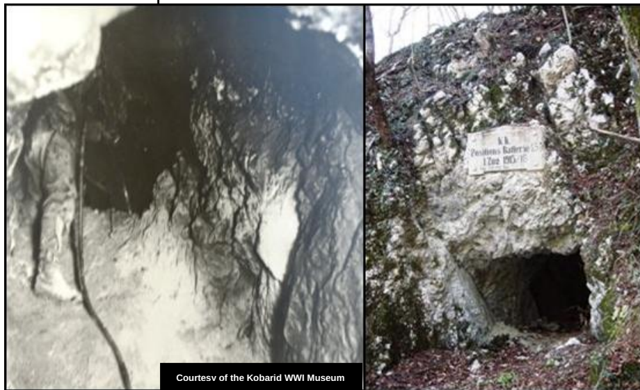
Figure 13. Austrian forces dug deep caverns, kavernen , into the mainly limestone geography throughout the Isonzo Valley. The limestone caverns provided adequate shelter from Italian heavy artillery and the effects of the alpine weather.
