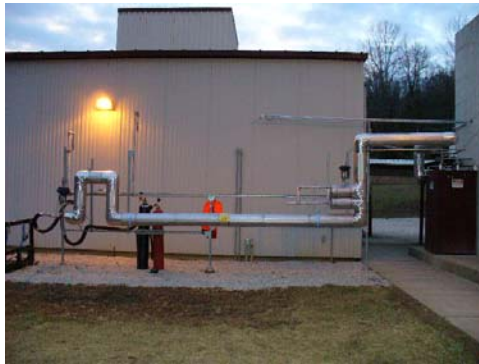
Figure 7: LOX supply line
