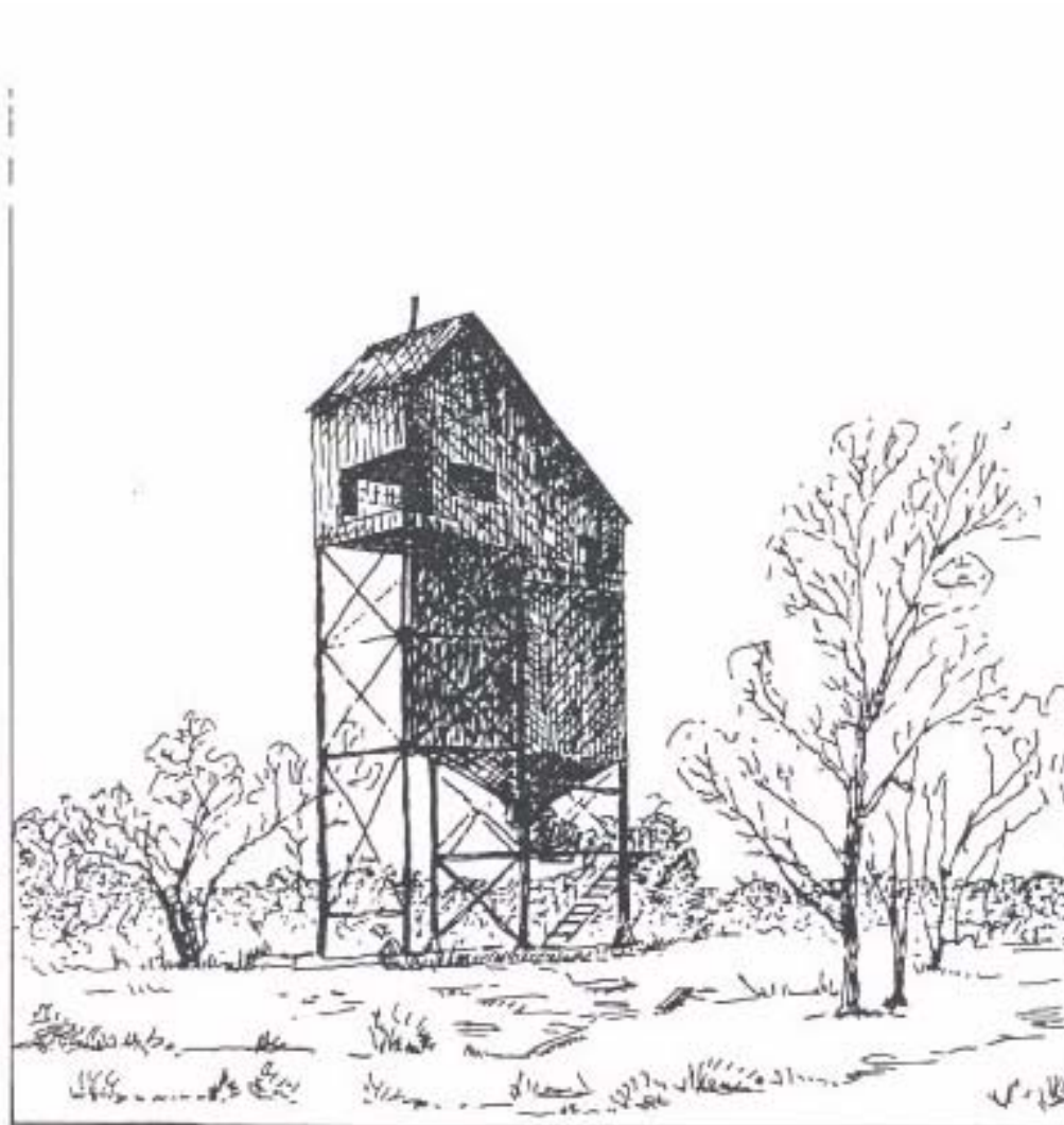
Ore loader in the Tar Creek area
