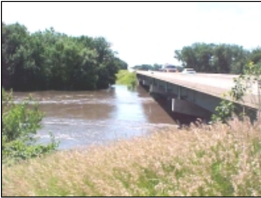
Downstream Side View (7/11/03)
