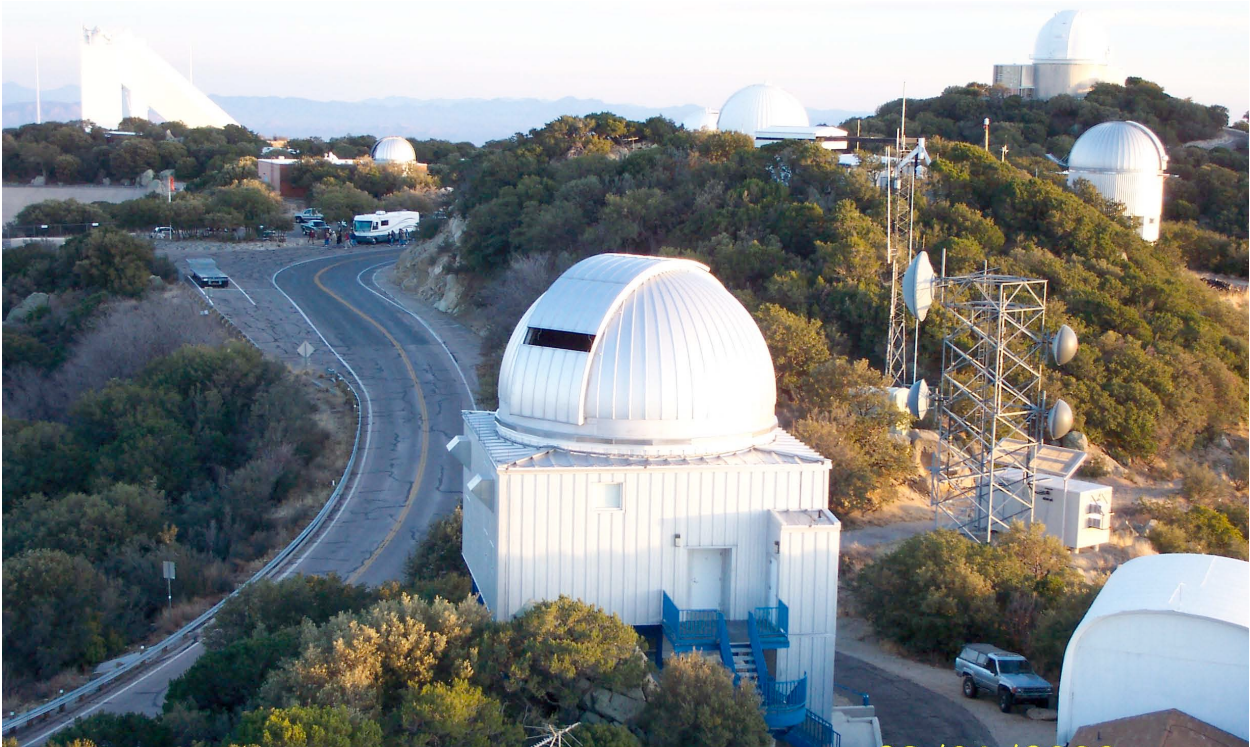
Figure 14: The 1.8 meter Spacewatch telescope located at Kitt Peak National Observatory, outside of Tucson, Arizona. It is a f/2.7 telescope (meaning that the ratio of the focal length of the telescope to its aperture, or diameter, is 2.7) with the CCD placed at prime focus. Follow-up images of 2003 MW12 were made using this telescope, the first to be taken since its discovery 3 months prior, confirming the objects status as a valid Kuiper Belt object. Picture taken by Professor Jeffrey Larsen of the United States Naval Academy.
