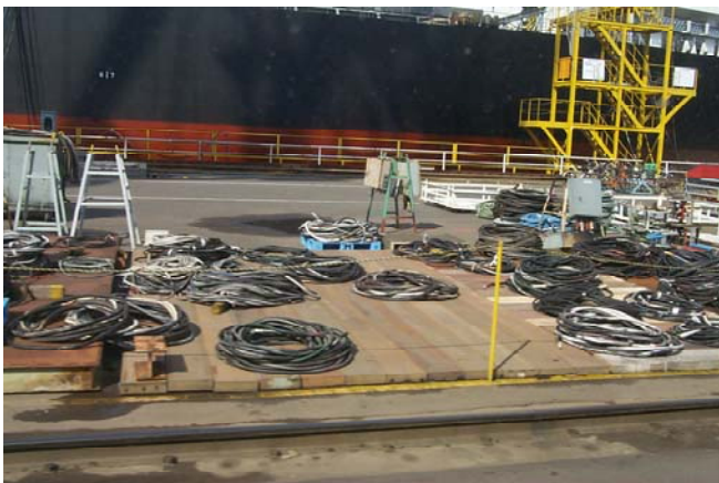
Photo 25: Wiring Cut to Length & Staged
