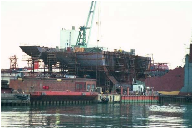
Photo 30: Turn-key Outfitting of Stern
