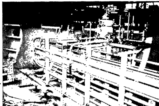
Figure 3.16 CLOSE-UP OF ENGINE ROOM -- IHI-KURE
