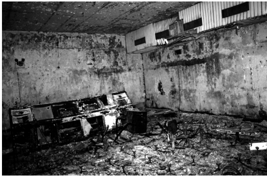
A destroyed underground bunker
