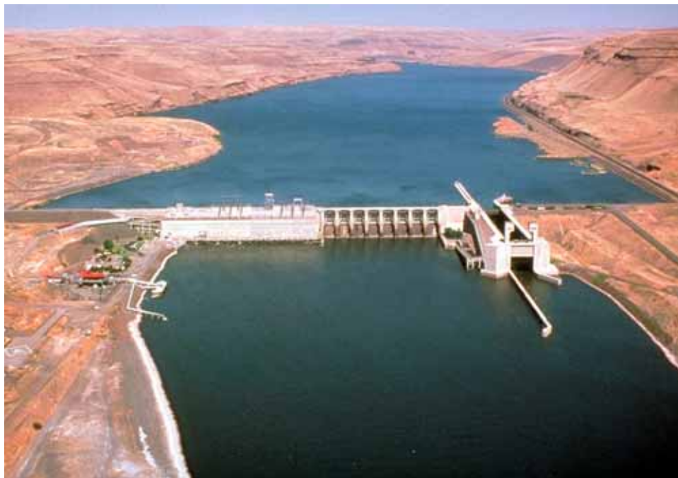
Figure 2. Lower Monumental Lock and Dam (forebay at top of photo)
