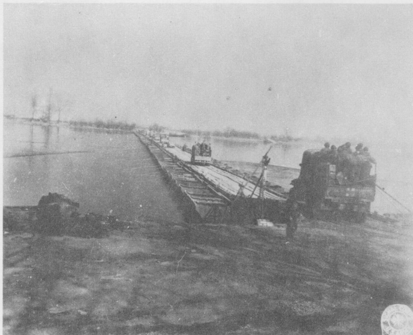
Photo No. 18 TRAFFIC ROLLS OVER HEAVY PONTON BRIDGE AT NIERSTEIN.
