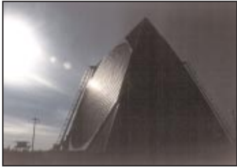
■ The PAVE PAWS radar network system.
