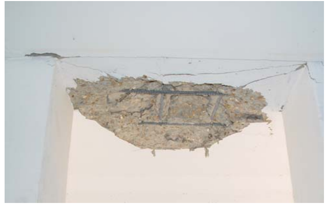
Figure 15. Internal spall surface from Round 1
