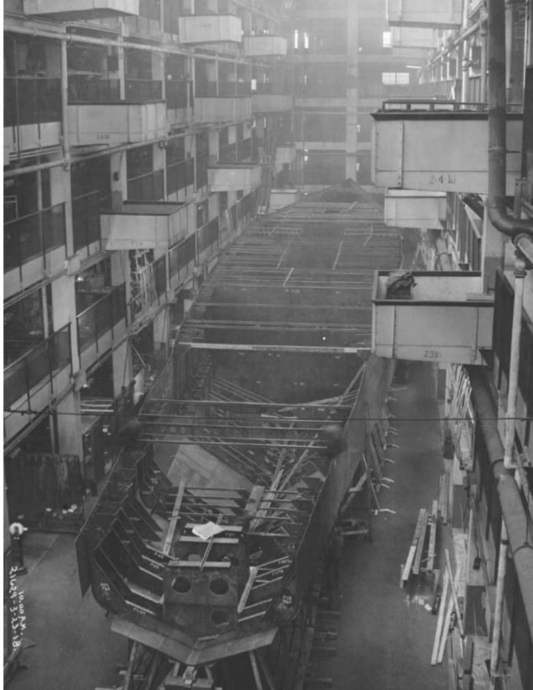
Figure 24: Main Eagle Boat Assembly Building (“Bldg. B”), River Rouge Plant 55
