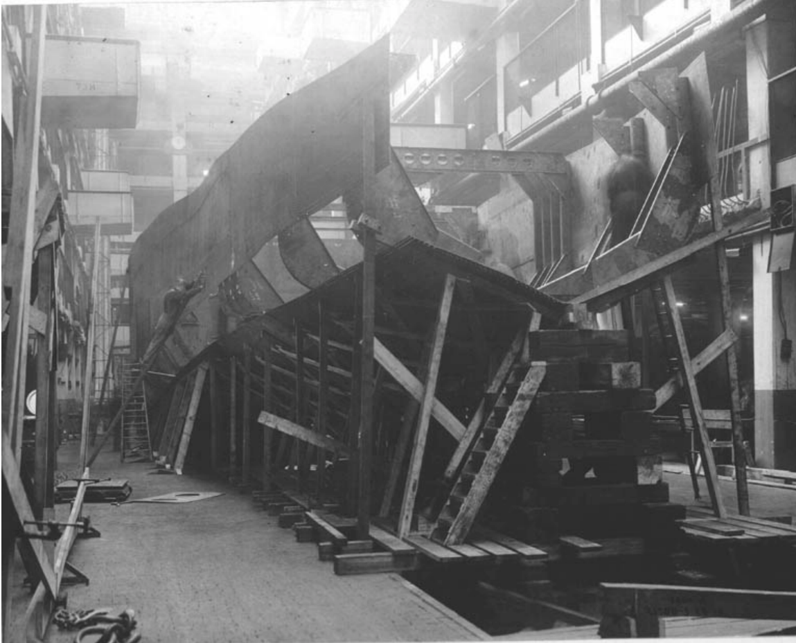
Figure 29: Hull Construction on Eagle Boats 62
