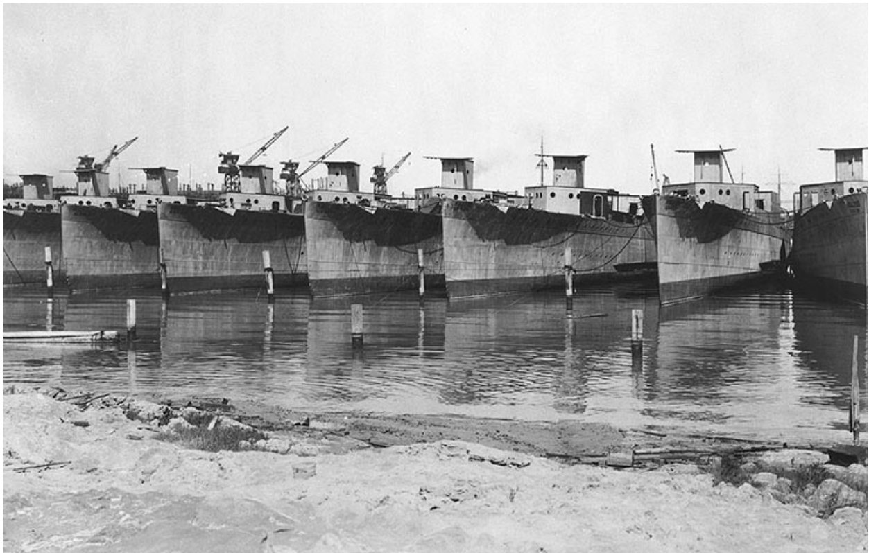
Figure 18: Destroyers fitting out at BethSF in 1920 33
