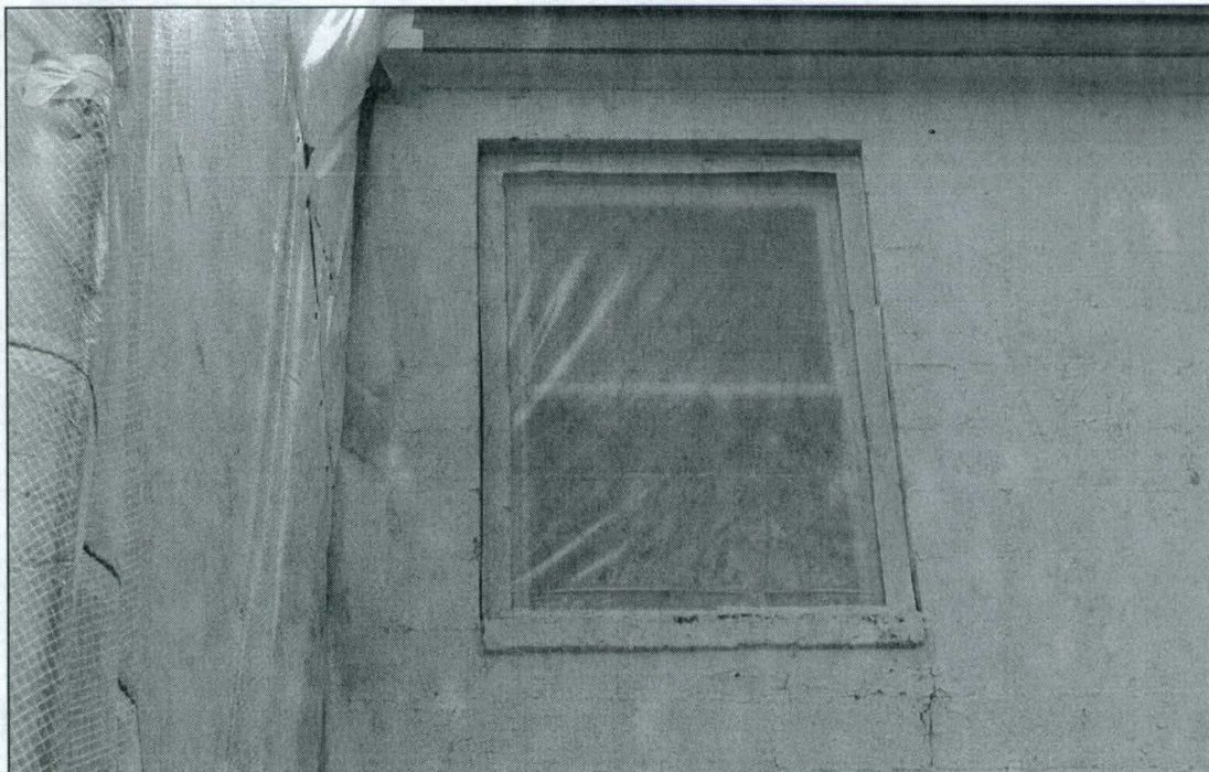
Figure 2. Critical barrier of 6-mil polyethylene sheeting placed over window.
