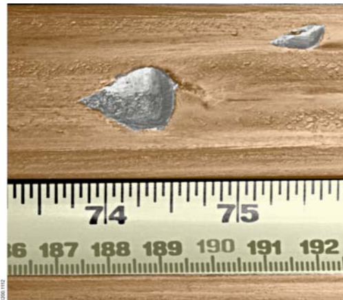
Figure 4.1. Gouging in Copper Rails (from Stefani, IAT)
