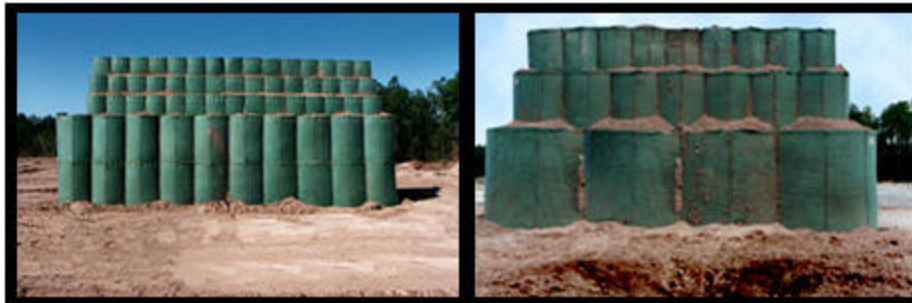
Figure 36. Wire Frame, Fabric-Lined Container/Concertainer Revetment.
