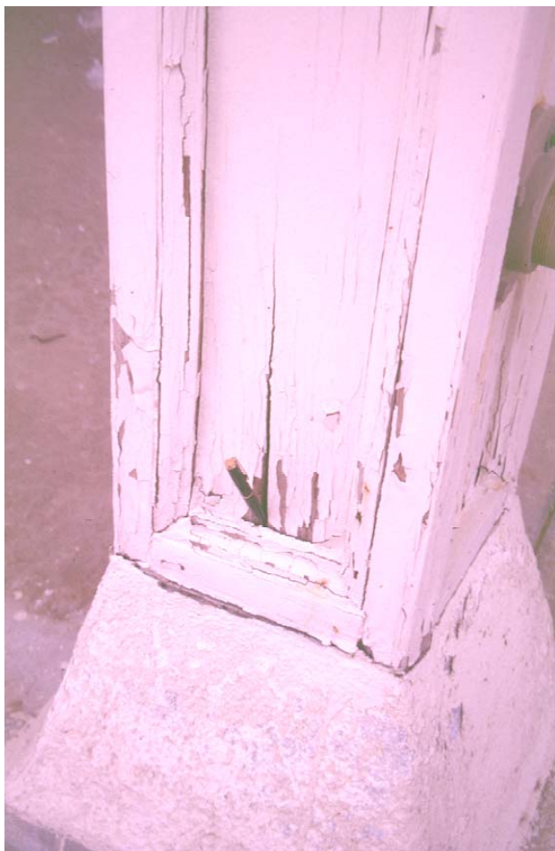
Photograph 78. Split trim work on Conference Center's porch columns.
