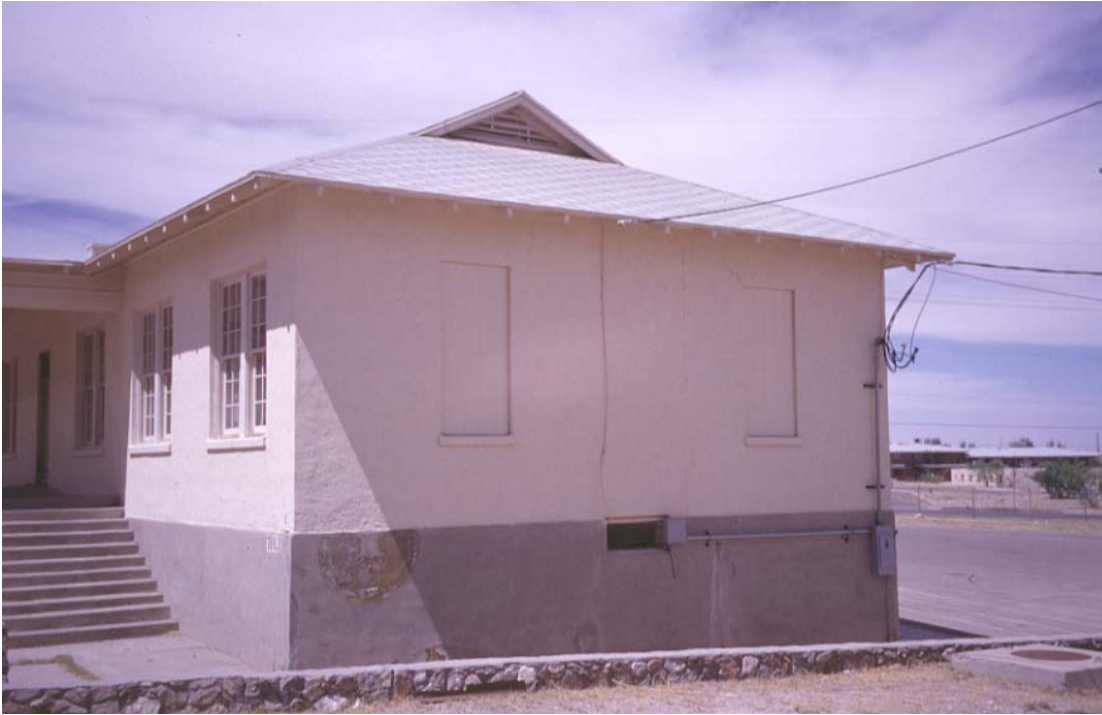
Photograph 80. Boarded windows in the south wall of Conference Center.
