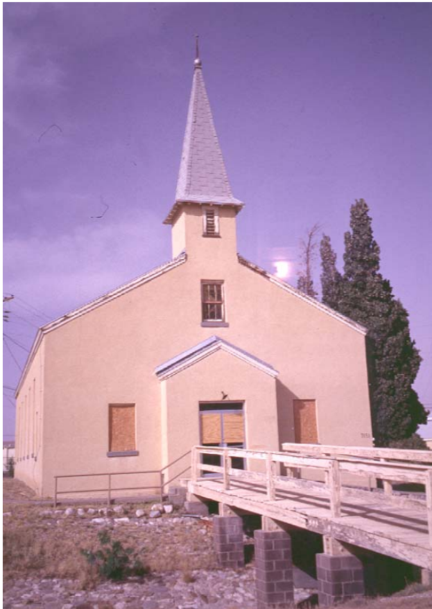
Photograph 6. Exterior photograph of Building 7151 (chapel).
