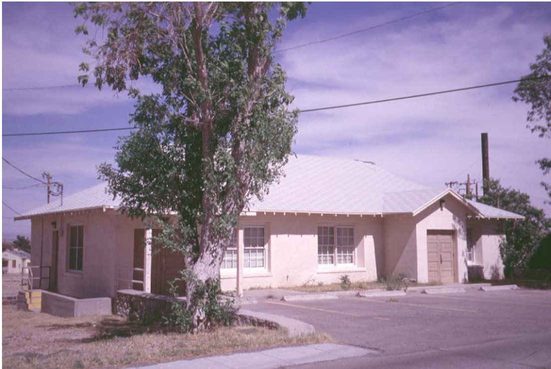
Photograph 60. Exterior photograph of Building 7166 (BOQ).
