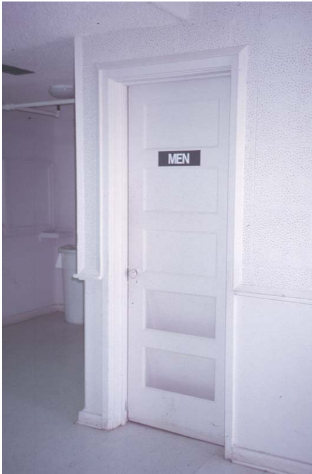
Photograph 18. Theater washroom door vent detail.
