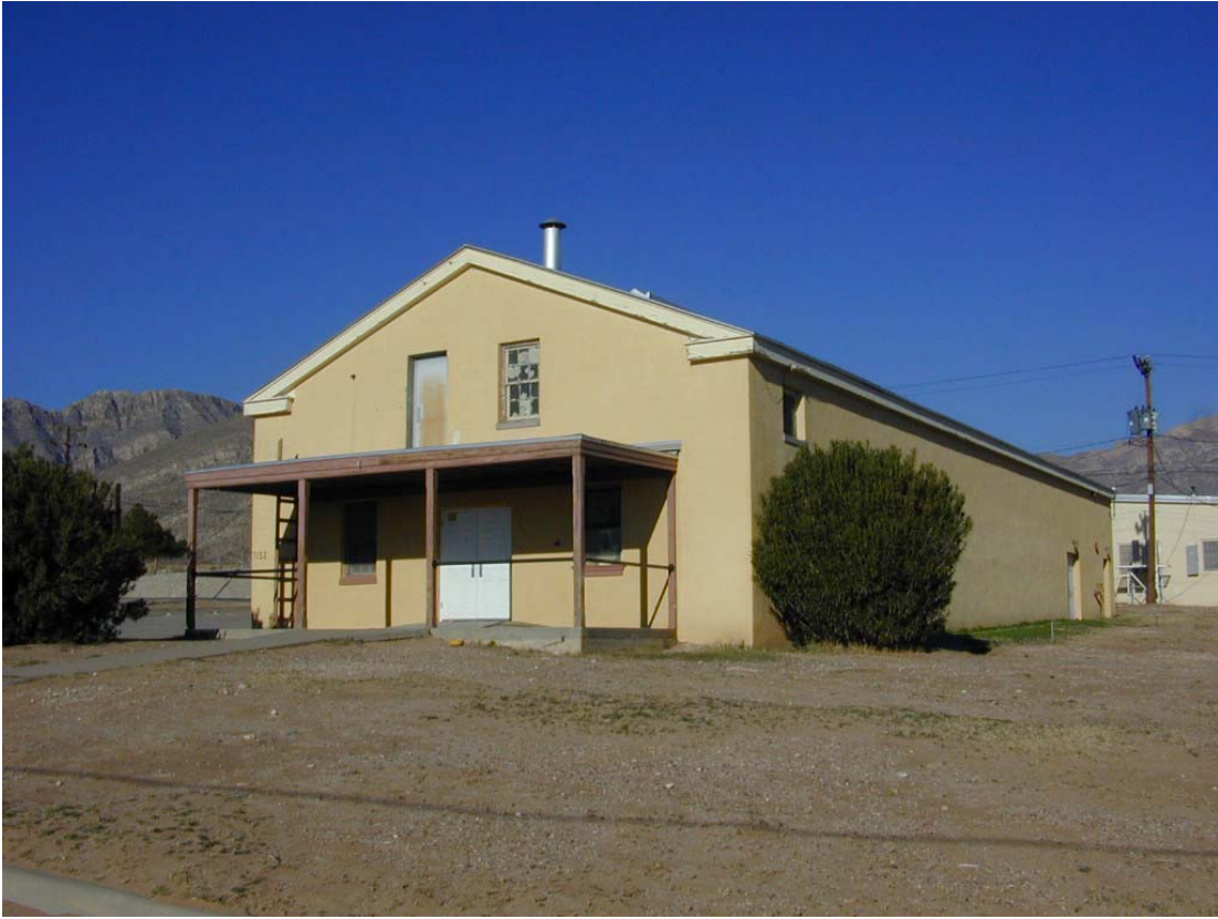
Photograph 15. Exterior photograph of Building 7152 (theater).
