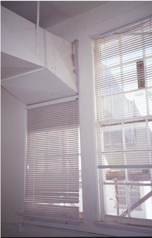
Photograph 59. Non-historic modification of window sashes in Building 7159.
