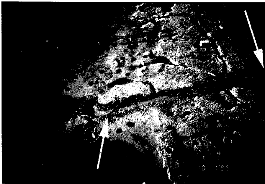
Figure 5. Bread Truck ditch, October 1996. Arrows point to the ends of the blasted ditch. Headwall erosion is evident to the left of the left arrow.
