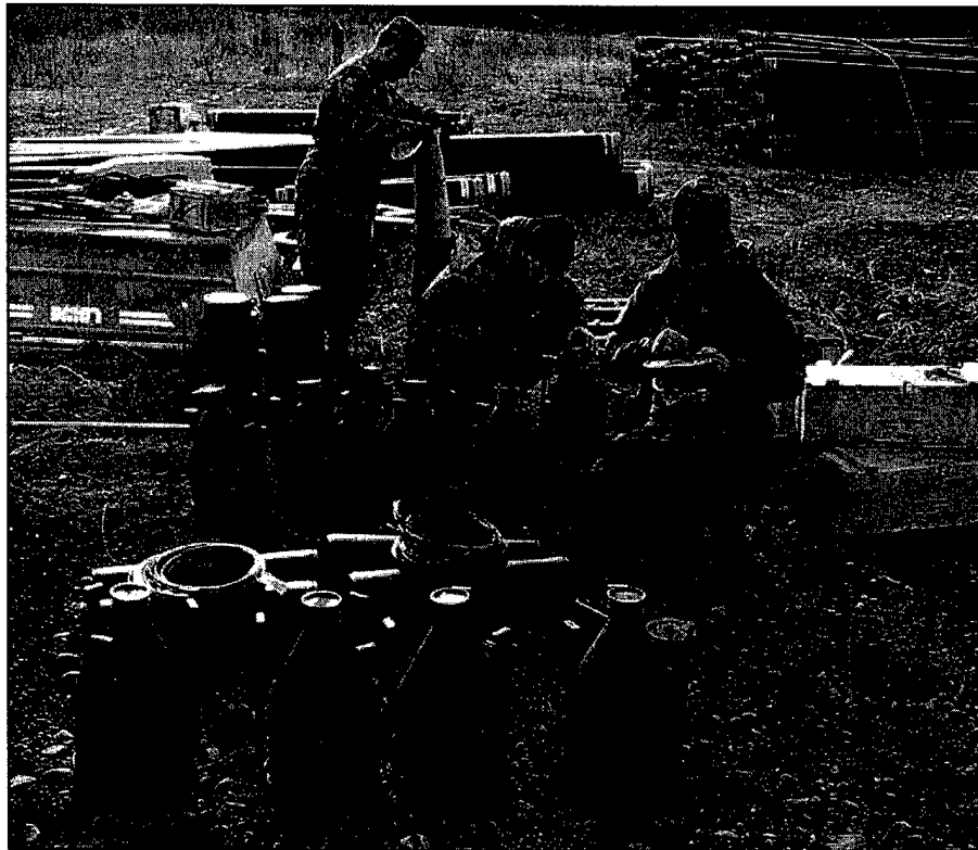
Figure 4. Preparation of shaped (foreground) and cratering charges.
