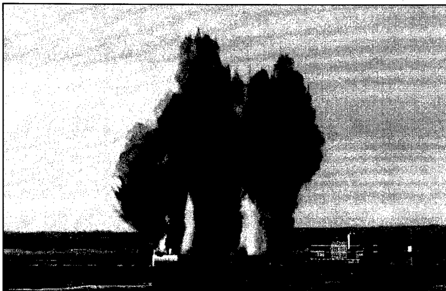
Figure 10. Blasting a sump drainage ditch with Bangalore torpedoes and det cord.
