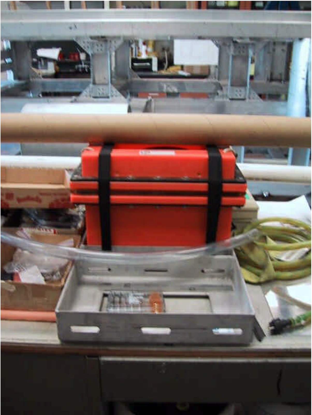
Figure MED-48: Battery Straps and Battery in Tray. (tilted view)
