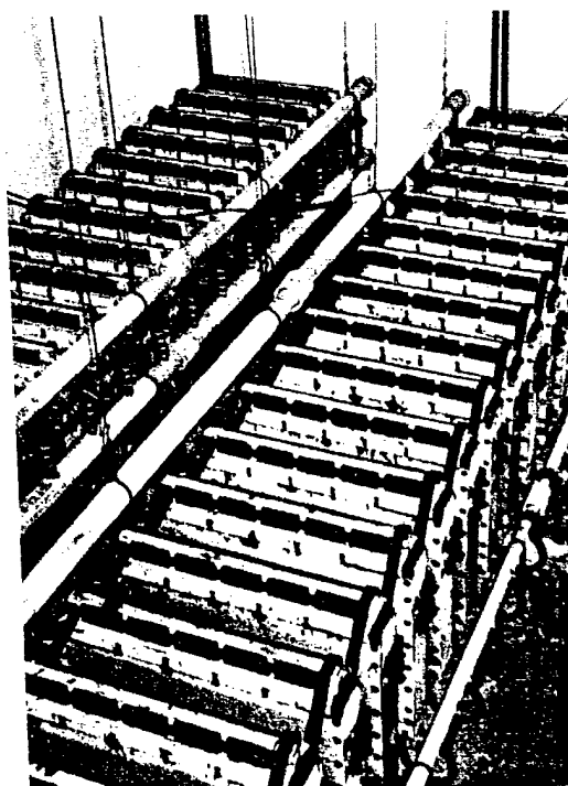
Figure 2. Los Angeles KClO 3 Production Plant 800 Amp Electrolytic Cells
