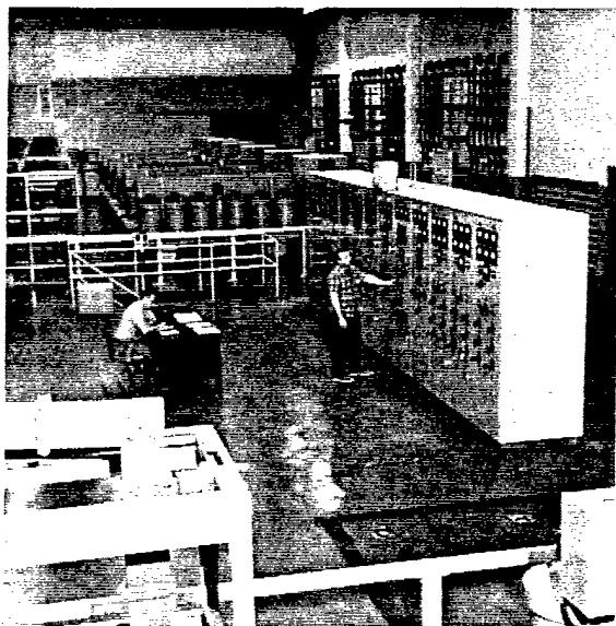
Figure 11. Mercury Arc Rectifiers and Controls Henderson, Nevada Plant
