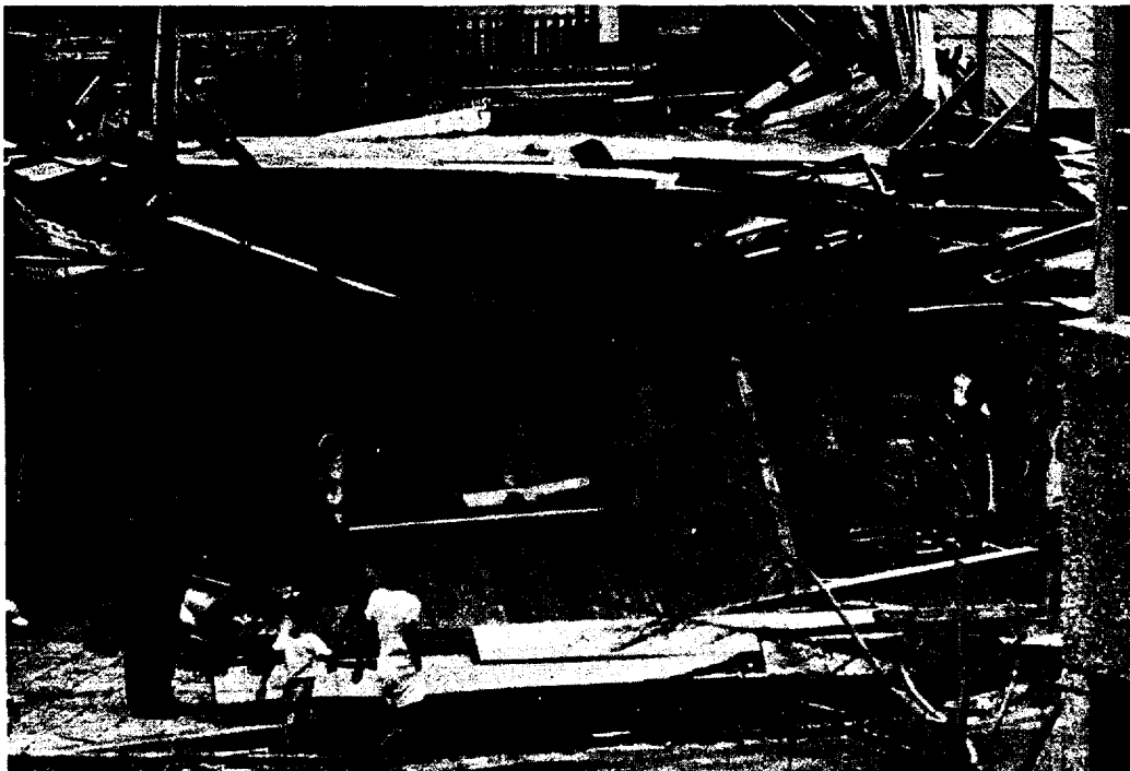
STRUCTURAL DAMAGE, NAHA, OKINAWA. NOTE INVERTED ROOF, CEILING AND SUPPORTS RESTING ON ROOF OF SHOP. SEPTEMBER 1961. (PACIFIC STARS AND STRIPES)
