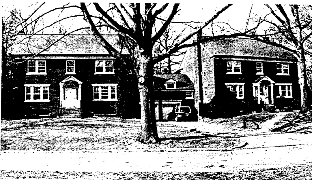
Figure 36. Lee Gate area houses built in the 1930s.
