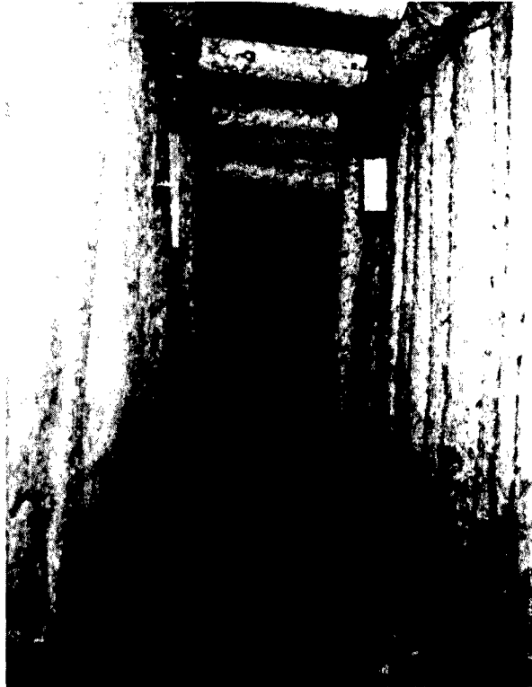
Figure 3.7 Looking down the Horizontal Part of the Entryway into the Main Room of Half-Scale Small-Pole Shelter LN316-1A. Note the slight inward bowing of the wall poles. The vertical post extended down 2 feet through the refilled earth to bedrock; its top, before being sawed off, held the Beam Deflection Gauge.
