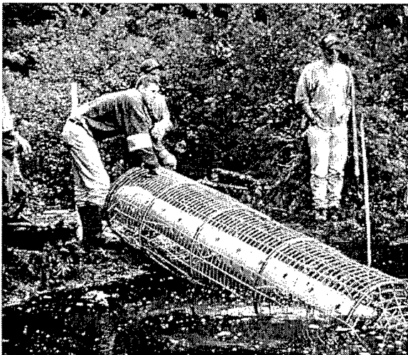
Figure 5. Clemson leveler intake pipe
