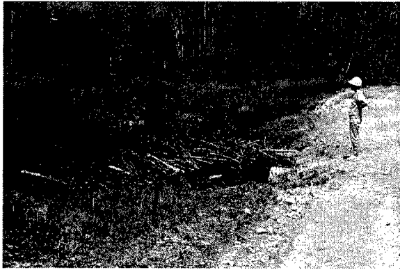
Figure 2. Pre-dam installed at culvert intake
