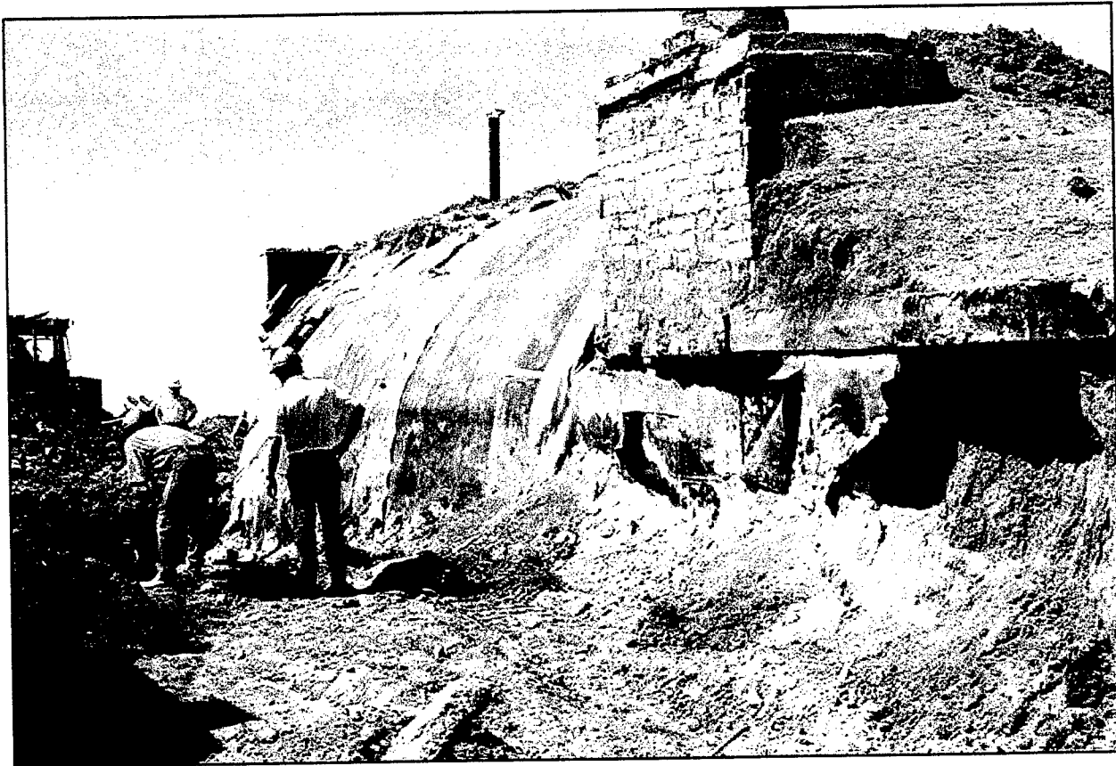
Figure 33. Bermed storage facility being exhumed for destruction and disposal. A black tar paper-like material covers the reinforced concrete. Derzhavinsk, Regiment 2, Silo 3.
