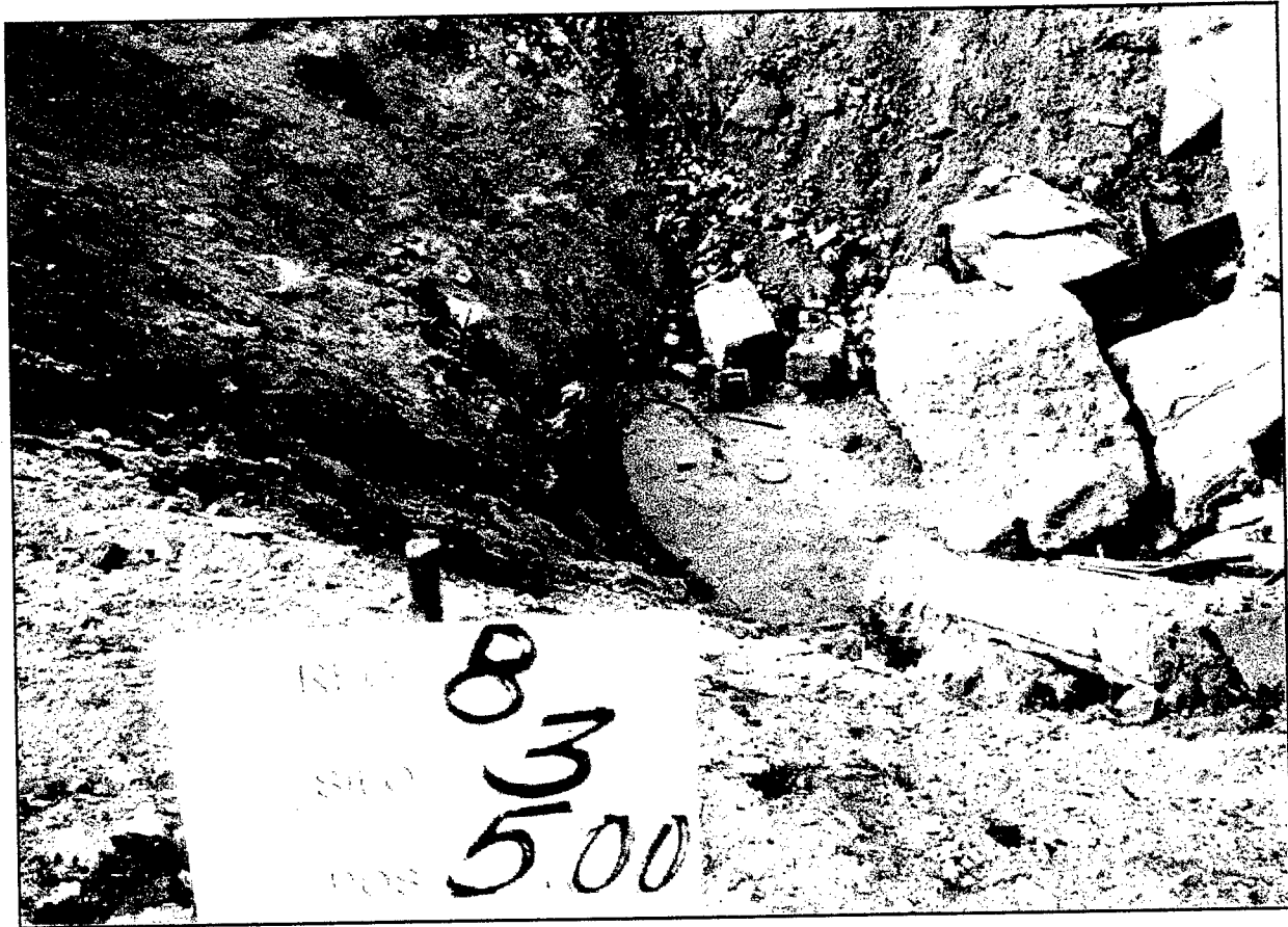
Figure 43. After the silo tube has been capped, additional rubble is pushed into the crater over the cap. Zhangiz Tobe, Regiment 8, Silo 3. Courtesy of Brown & Root/ABB SUSA.
