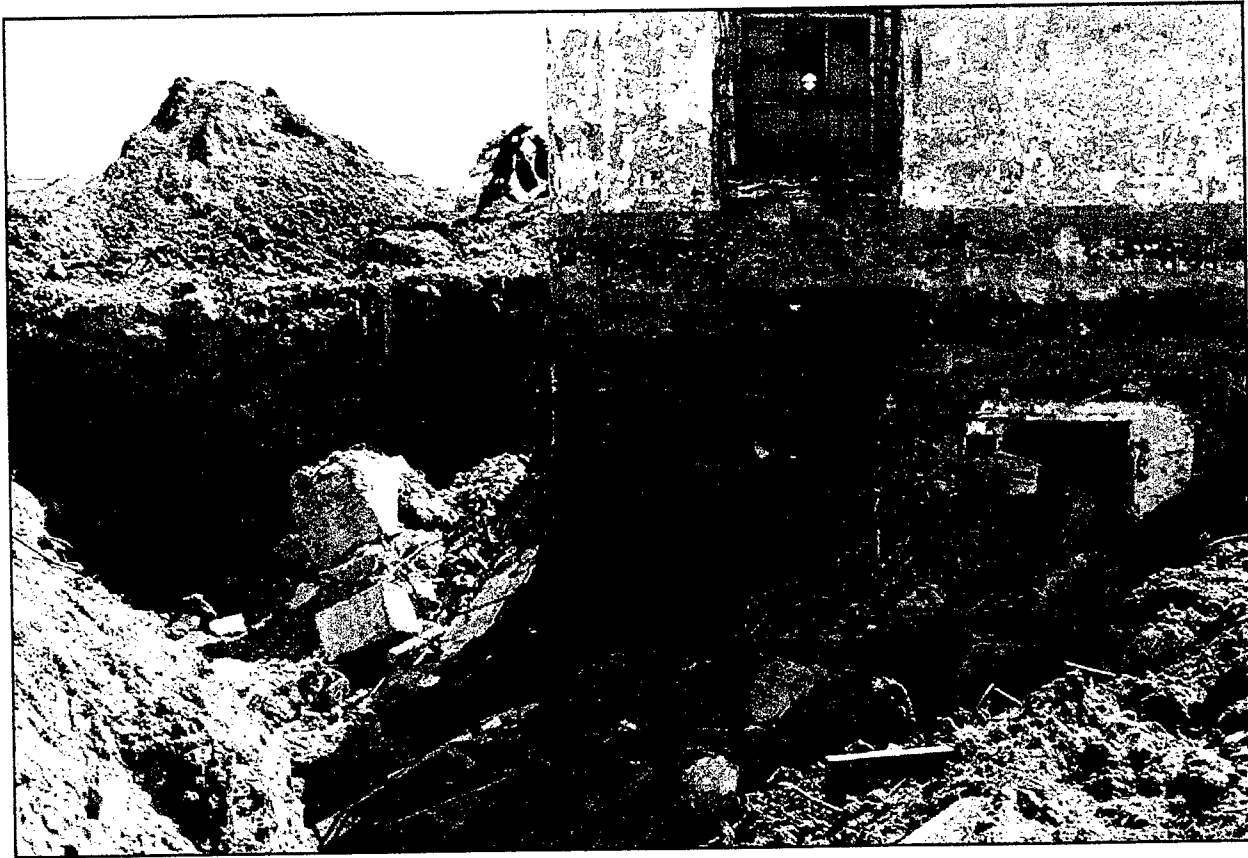
Figure 47. A pit has exposed the subterranean section of the "Force Protection" security building. The pit is partially filled with building rubble. Derzhavinsk, Regiment 2, Silo 2.
