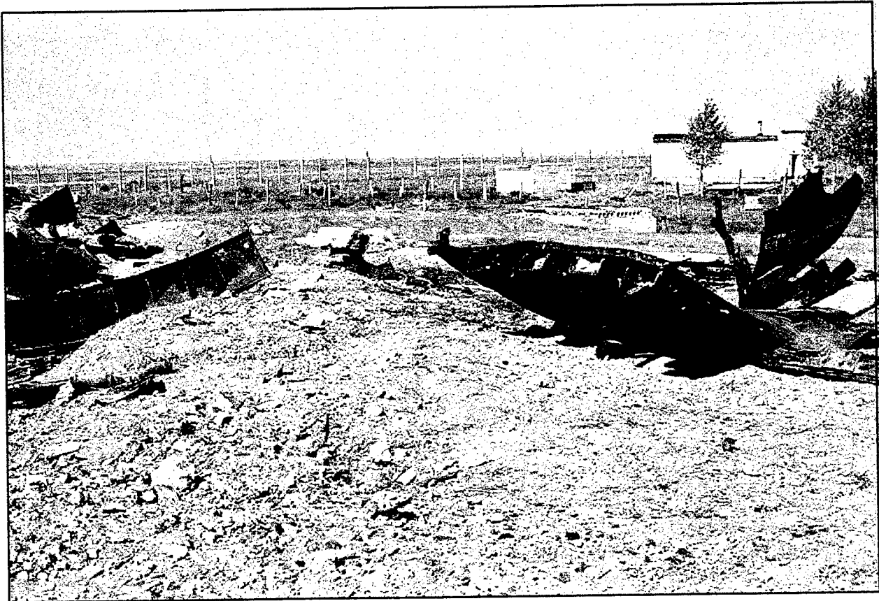
Figure 8. Metal and concrete debris on the crater rim. The ribbed metal plate on the right may be part of the headworks wall. The transformer substation is in the right background. Derzhavinsk, Regiment 2, Silos 5/7.
