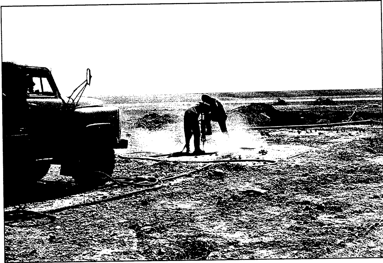
Figure 39. Drilling dynamite emplacement holes in the two-meter thick reinforced concrete support blocks of the transporter loading ramp. Derzhavinsk, Regiment 2, Silo 2.
