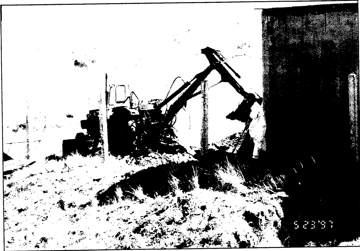
Figure 35. Abatement contractor crew removing PCB contaminated soil near a transformer building. Zhangiz Tobe. Photo courtesy of Brown & Root/ABB SUSA.
