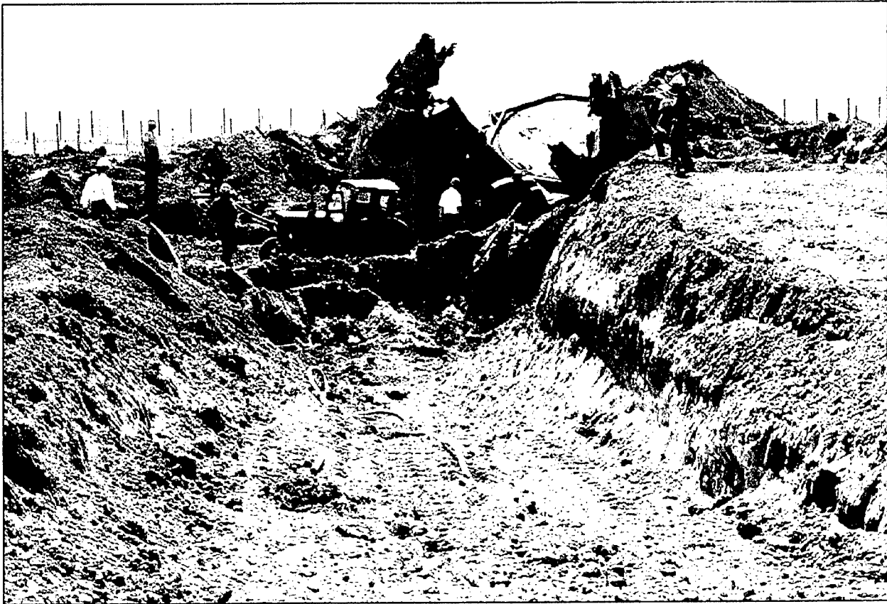
Figure 40. Ramp partially dug down to the silo crater for removal of metal and concrete, and backfilling of the silo tube with debris. The silo door pocket is on end. Derzhavinsk, Regiment 2, Silo 4.
