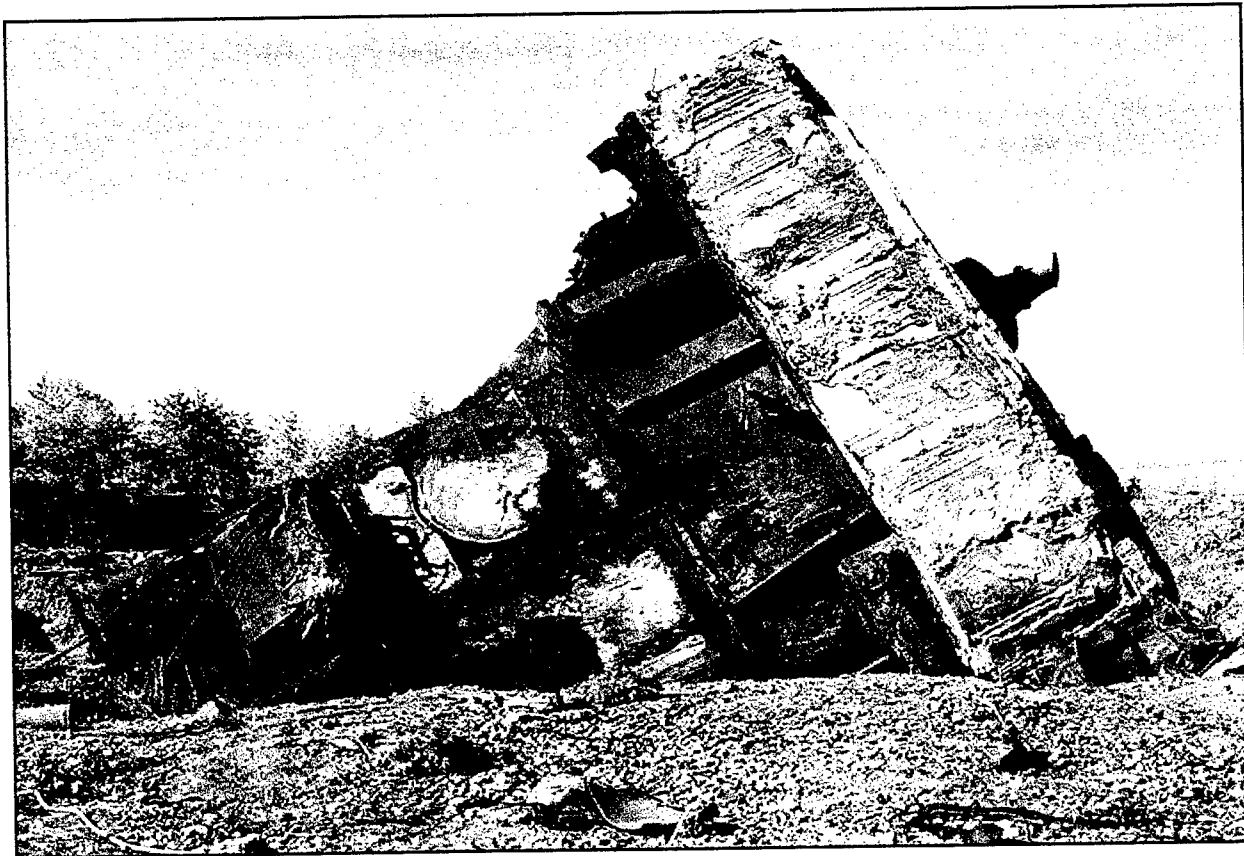
Figure 37. Relatively intact LCC silo door pocket still attached to part of the headworks wall. Derzhavinsk, Regiment 2, Silo 7.
