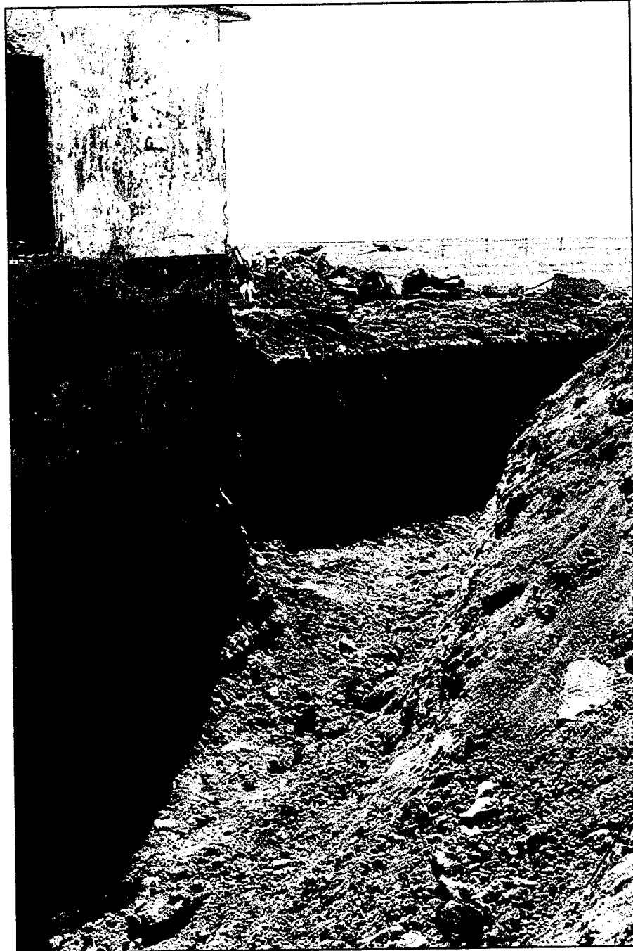
Figure 21. Trenching along side the "Force Protection" security building has exposed the subterranean level of the building and the associated shallow buried tunnel. The buried structures are lined with red clay brick. The excavation is about three meters deep in dry fine-grained silt and clay. Derzhavinsk, Regiment 2, Silo 2.
