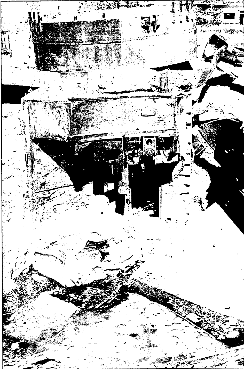
Figure 16. Underground tunnel entrance into the LCC silo headworks revealed in the crater. The round silo door rests on the crater rim. Derzhavinsk, Regiment 2, Silo 7.
