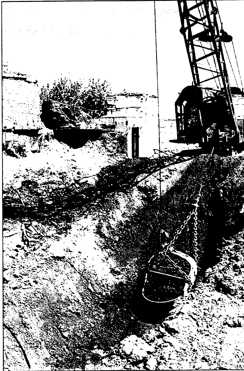
Figure 46. Excavating a pit along side a bermed storage bunker for the disposal of the bunker. The earth is brown, fine-grained silt and clay; the gray-white material is poorly sorted sand, possibly dumped in place during construction. Derzhavinsk, Regiment 2, Silo 3.
