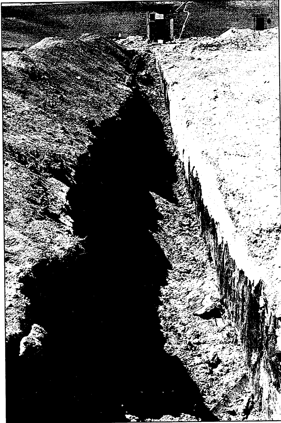
Figure 15. Partially excavated shallow buried tunnel between the cooling system building (in background) and the Launch Control Center (LCC) silo. Derzhavinsk, Regiment 3, Silo 7.
