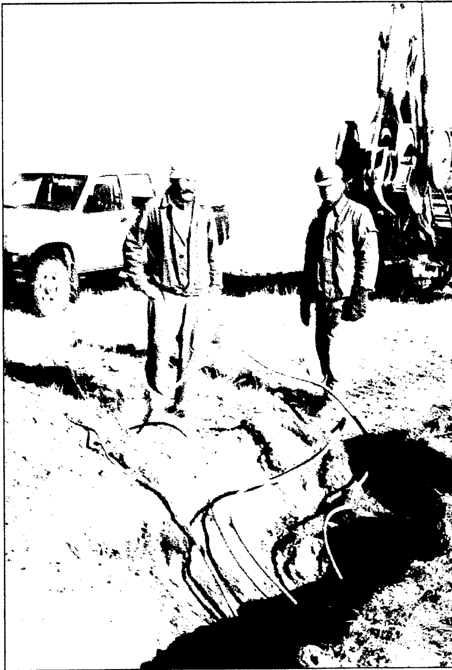
Figure 48. Cable salvaging operations. Four cables are being retrieved from one trench. Zhangiz Tobe. Courtesy of Brown & Root/ABB SUSA.
