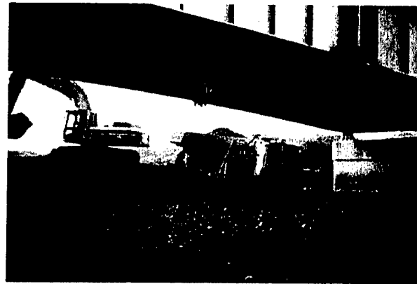
Channel management activity required additional heavy equipment in the immediate area of the Wilson Bridge. Aggradation of material was so excessive that the riverbed was lowered up to thirteen feet in this area. A small bulldozer was used to push the material out to the backhoe so that it could be loaded into the dump trucks
