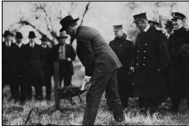
Secretary Daniels breaks ground for Building 1 in 1920.
