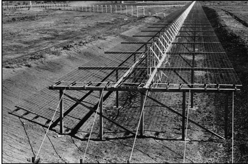
A series of surveillance transmitting antennae like this one at Lake Kickapoo, Texas, comprised a surveillance system developed by NRL to detect unannounced radio-silent satellites passing over the United States.
