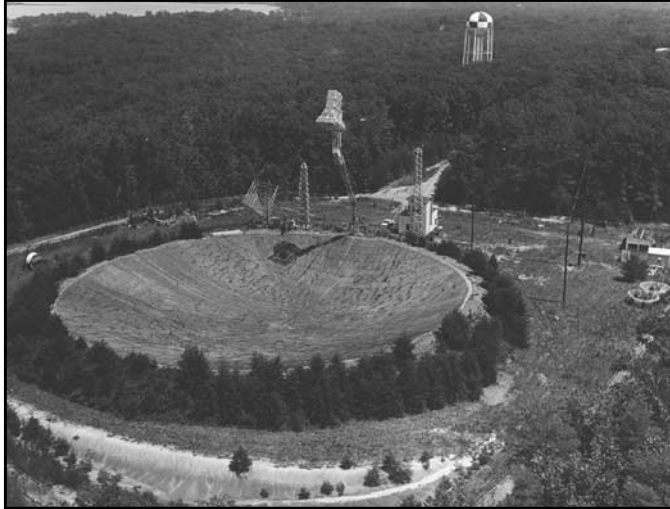
NRL built and used this 220-ft by 263-ft antenna in Stump Neck, Maryland, as part of a long-distance communication circuit involving Earth's natural satellite, the Moon, as the reflector of signals from the sender to receiver.
