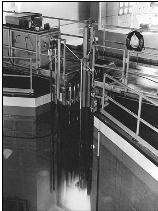
The core assembly of NRL’s research nuclear reactor, which first hosted chain reactions in 1956, is shown suspended in a pool of shielding water.
