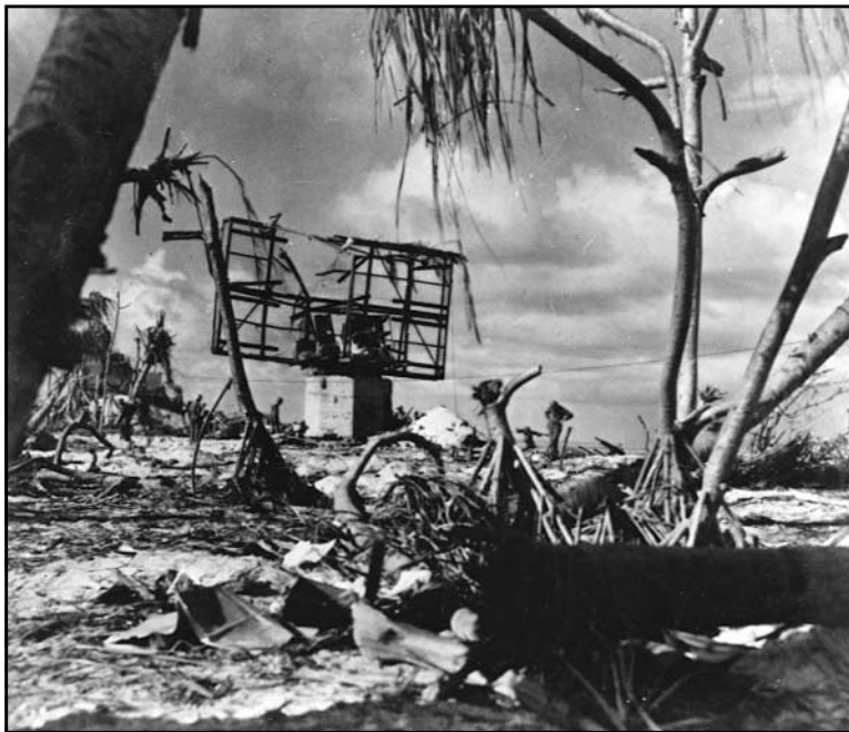
The remains of Japanese radar installations like this one were sent back to NRL for analysis and the development of countermeasures.
